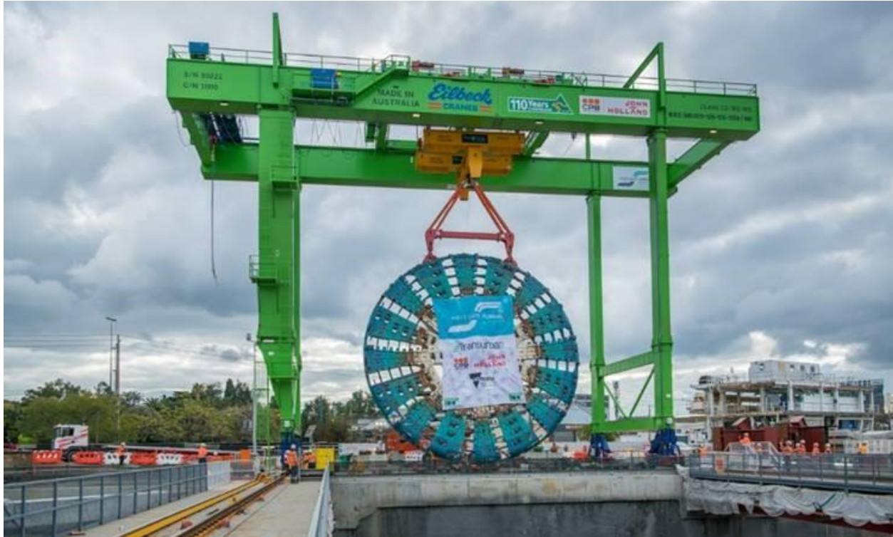
Gantry Crane delivering shield at project commencement
