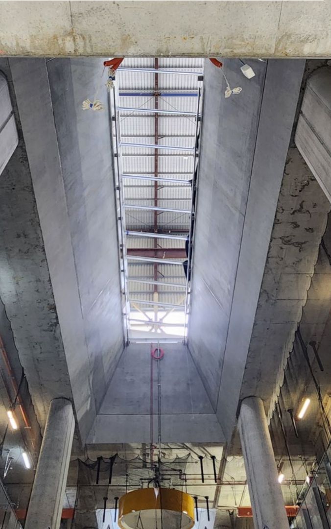
Skylight precast panels installed
