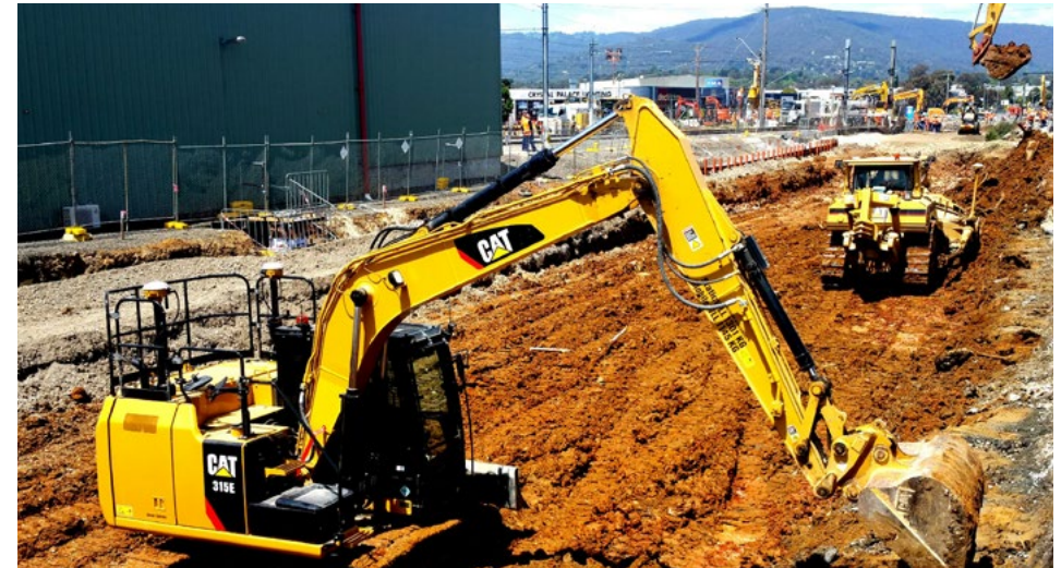
Asphalt works Scoresby Road
