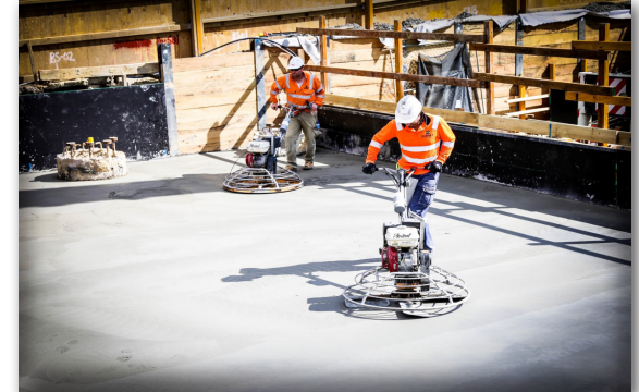
Concrete placed into bridge deck
