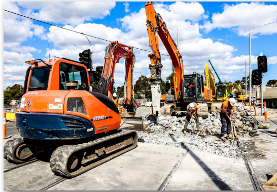
Excavation of Burke Road for the bridge deck
