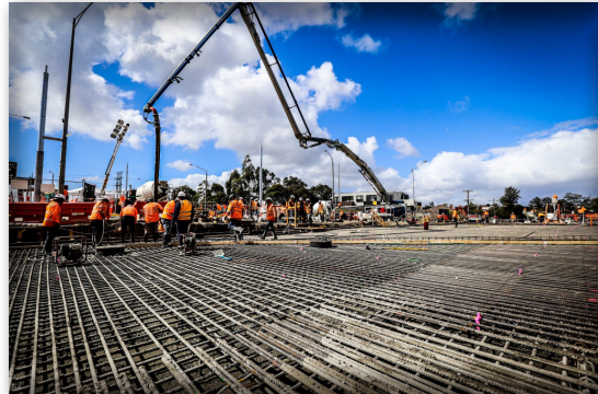
Steel reinforcement tied into Burke Road bridge deck
