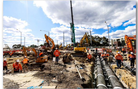
Installation of services in Burke Road
