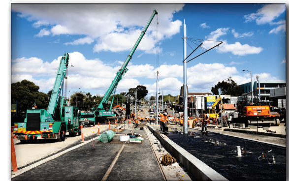
Realignment of tram line and construction of tram stop
