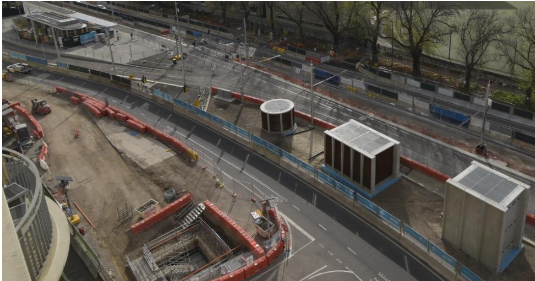
Back filling over station roof
