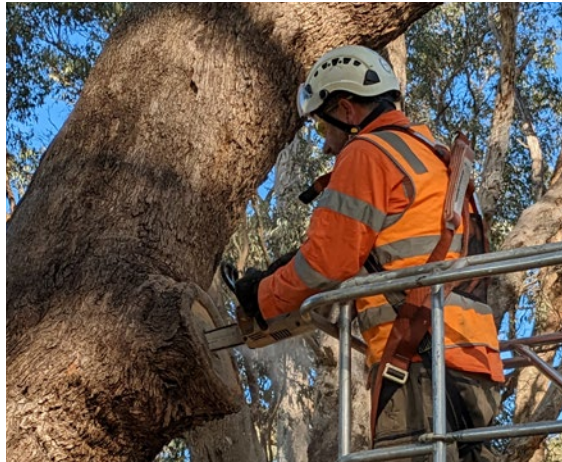
Figure 6: A hollow being drilled
