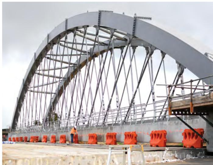
**1** | With all the steel arch segments in place, we installed and tensioned 76 steel bridge hangers to hold the bridge together.
