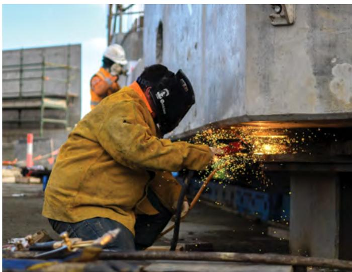
**2** | We then removed some of the temporary towers and bridge support structures.
