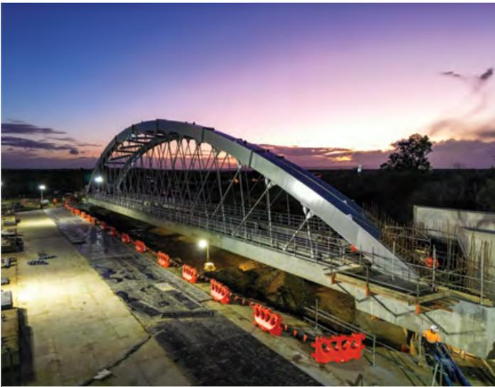
**6** | Moving at just 0.0008 km/h, it took two days to slide the 3,200-tonne rail bridge 27 metres into place over the rail line.
