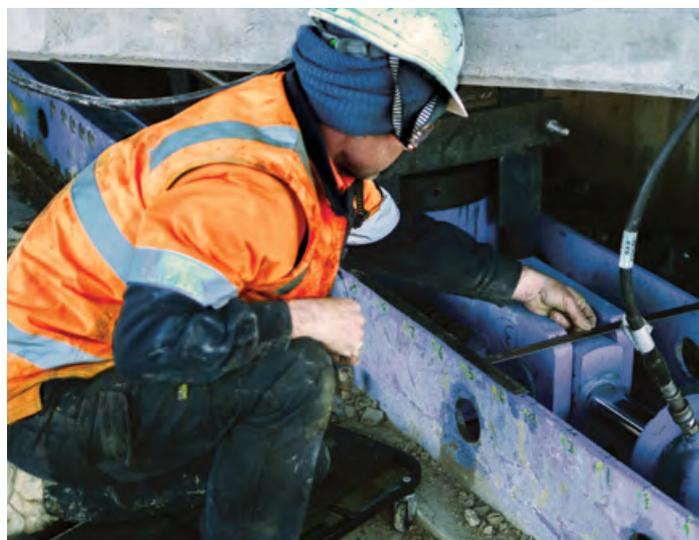
**3** | We installed a jack and sledge system underneath the bridge that would slowly lift and push it into its final resting place.
