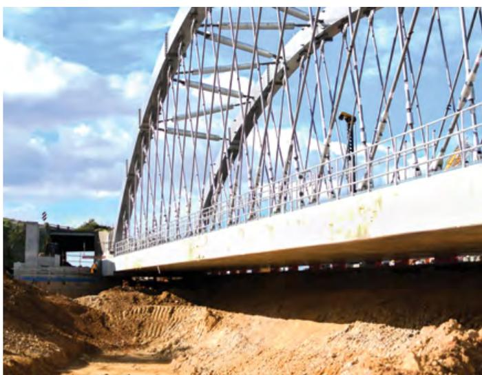
**4** | To make room for the bridge, we had to dig out more than 18,000 tonnes of material from the existing rail line and surrounding area.
