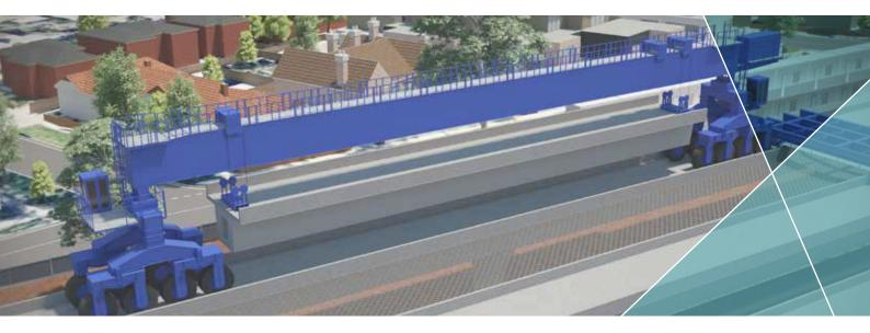
Due to the narrow rail corridor between Grange Road, Caulfield and Poath Road, Hughesdale, specialist equipment, including two gantry cranes and a straddle carrier, will be used to construct the elevated rail line.
