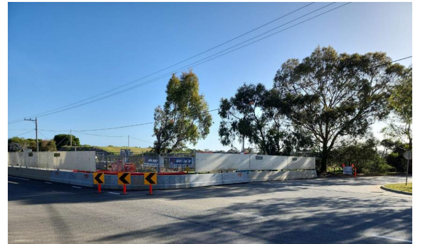
Images: Site investigation works along Old Dandenong Road
