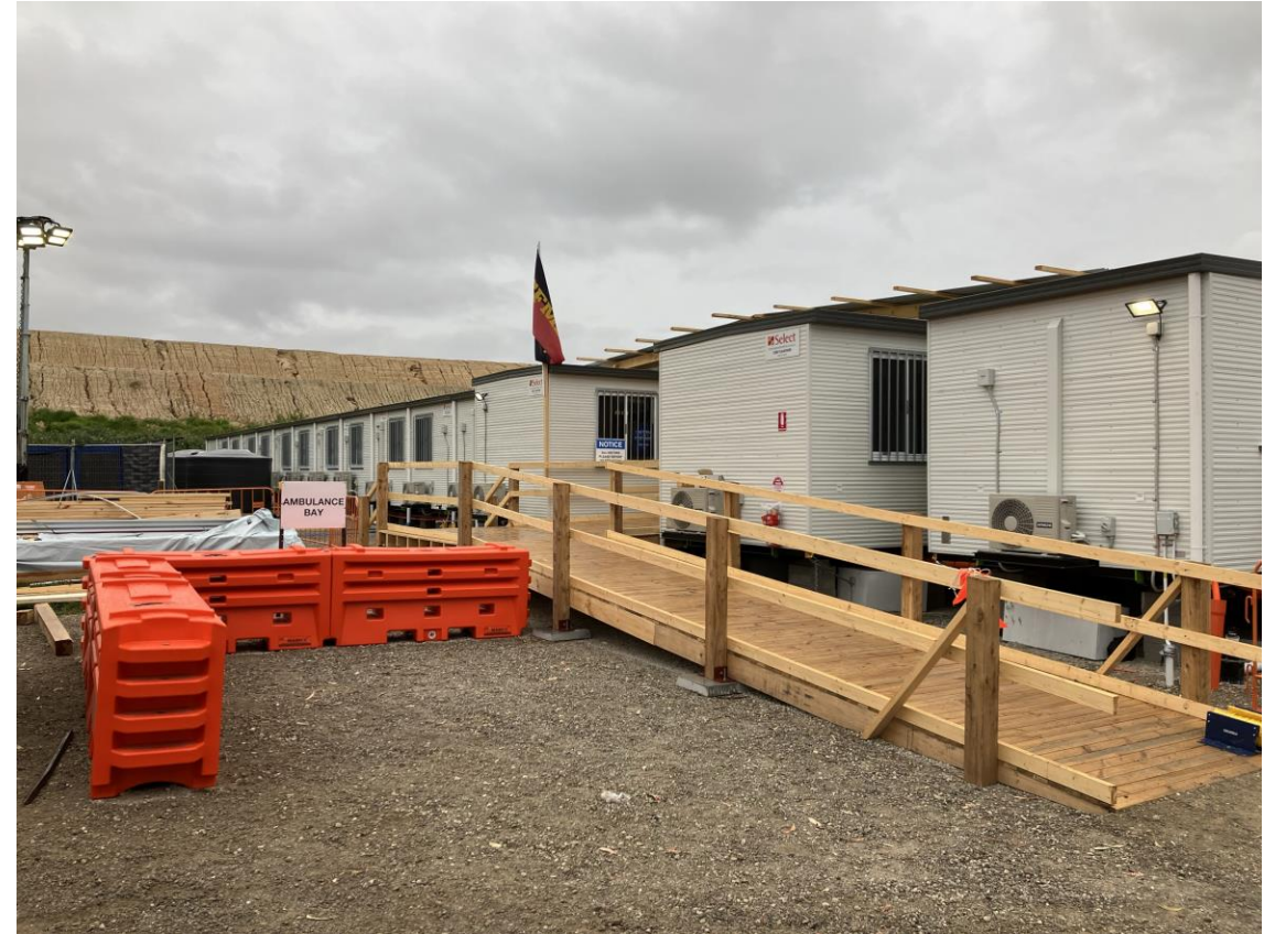
Image: Permanent site facilities at 217 Kingston Road
