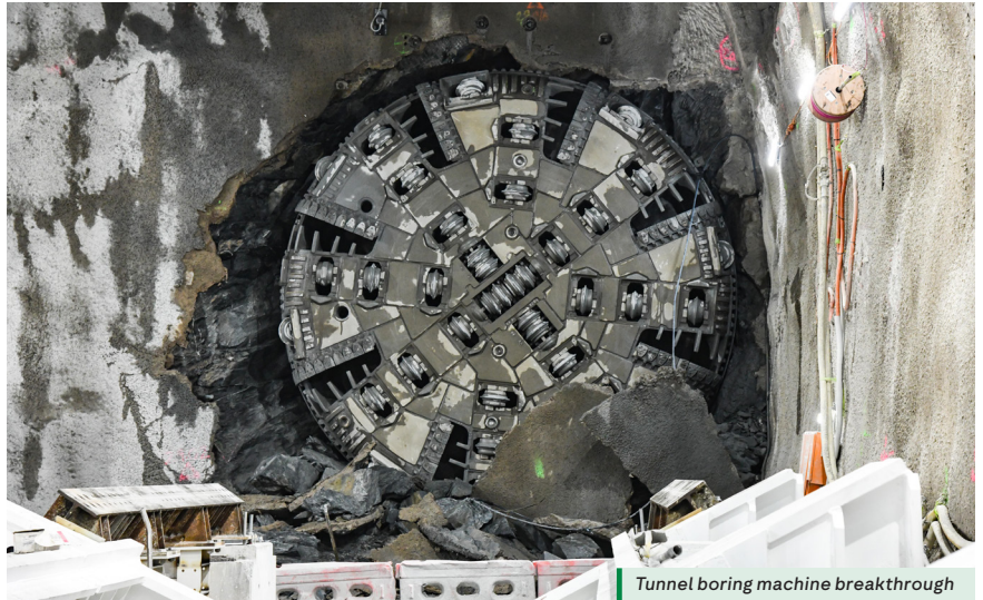
Tunnel boring machine breakthrough
