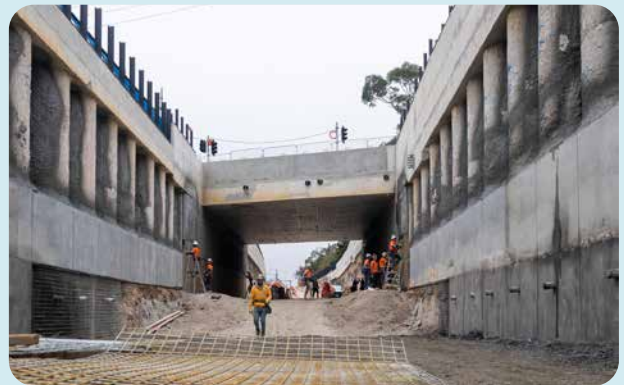
561 piles have been installed to support the new rail trench.
