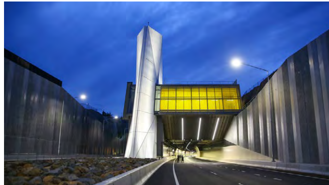
FIGURE 21 Demonstrates: integrated ventilation structure and tunnel approach. Waterview Tunnel, Auckland. Design: Warren and Mahoney, Image: NZ Transport Agency
