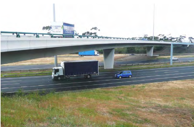
FIGURE 5 Demonstrates: a continuous and streamlined pier and box girder bridge structure design. Image: VicRoads
