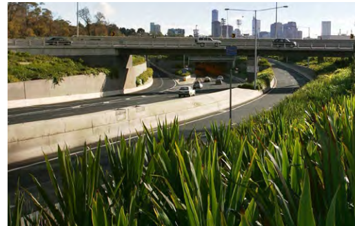
FIGURE 140 Demonstrates: a landscape design that responds to the high speed viewing environment through the use of terraced planting. CityLink, Melbourne. Design: EDAW, Image: GHD
