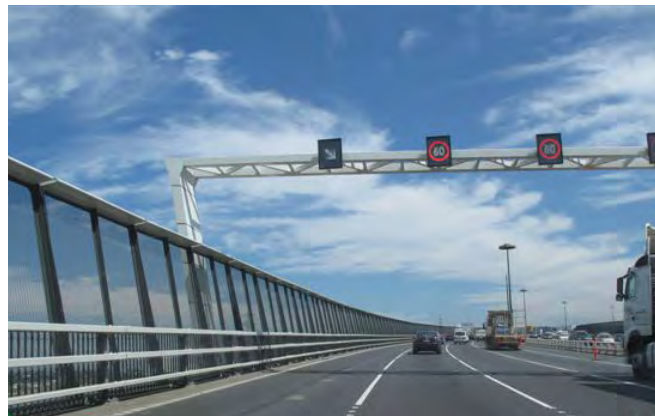
FIGURE 41 Demonstrates: Visually permeable safety barriers comprised of high quality architectural materials. Westgate Bridge, Melbourne. Design: Peter Elliott
