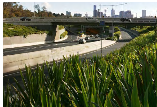
FIGURE 94 Demonstrates: a landscape design that responds to the high speed viewing environment through the use of terraced planting. CityLink, Melbourne. Design: EDAW, Image: GHD
