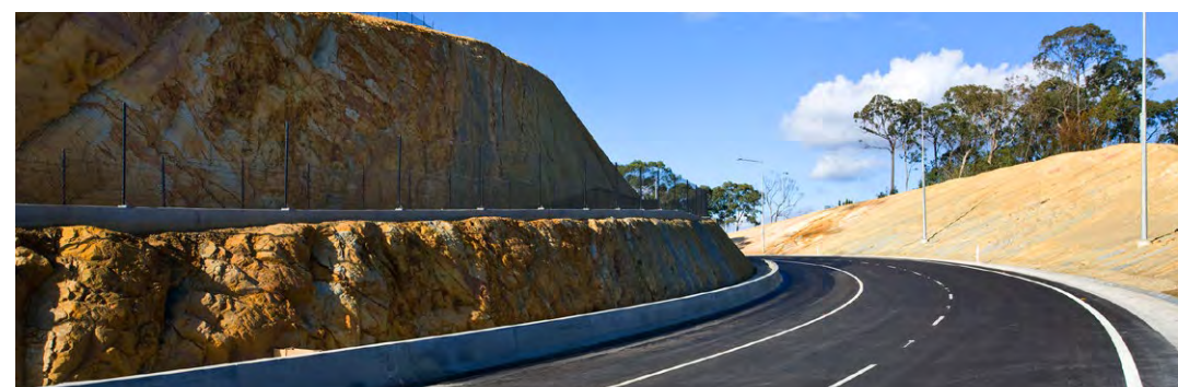
FIGURE 114 Demonstrates: use of existing natural stone in cutting as a design feature. EastLink Freeway, Melbourne. Design: Wood Marsh and Tract Consultants, Image: EastLink
