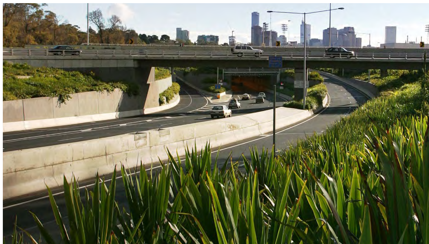
FIGURE 76 Demonstrates: a landscape design that responds to the high speed viewing environment through the use of terraced planting. CityLink, Melbourne. Design: EDAW, Image: GHD
