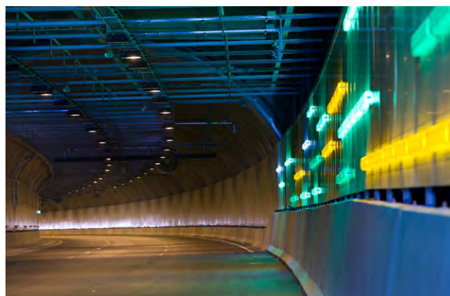
FIGURE 23 Demonstrates: Feature lighting used at strategic locations in tunnel to provide driver visual stimulation. EastLink, Melbourne. Design: Wood Marsh, Image: EastLink
