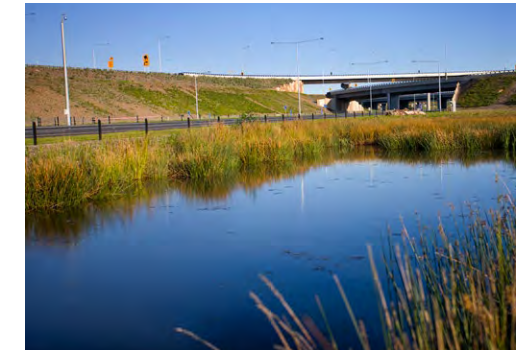
FIGURE 92 Refer Objective 4.3. Demonstrates: constructed wetland and vegetated embankment. EastLink, Melbourne. Design: Wood Marsh and Tract Consultants, Image: EastLink
