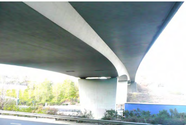
FIGURE 3 Demonstrates: continuous / smooth bridge underside and elegant soffit line. Western Ring Road, Melbourne. Image: VicRoads
