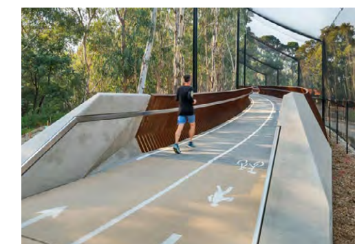
FIGURE 107 Demonstrates: integration of barriers and handrails. Darebin Yarra Trail, Melbourne. Design: VicRoads, Photography: Emma Cross
