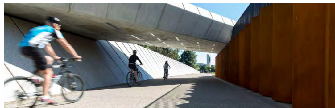
FIGURE 122 Demonstrates: use of natural light and a generous proportioned underpass. Bowen Place Crossing, Canberra. Design: Lahz Nimmo Pty Ltd and Spackman Mossop Michaels, Photography: Brett Boardman
