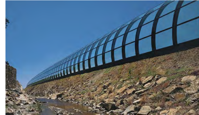
FIGURE 37 Demonstrates: semi-enclosed transparent noise wall to reduce visual bulk and allow light into the adjacent creek. Eastern Freeway, Melbourne. Design: Wood Marsh
