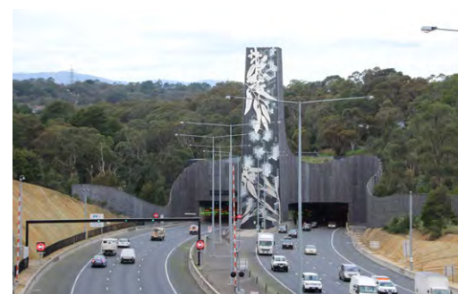
FIGURE 152 Refer Objective 1.5. Demonstrates: creative response and landmark feature that celebrates local context. Mullum Mullum Tunnel, EastLink, Melbourne. Design: Wood Marsh and Tract Consultants, Image: VicRoads
