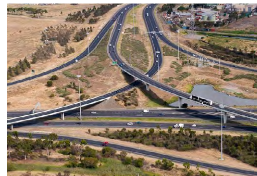
FIGURE 100 Refer Objective 4.3. Demonstrates: interchange acting as a navigational node with the integrated built form sensitively sited in the landscape. M80 / Princes Interchange, Image: Vic Roads
