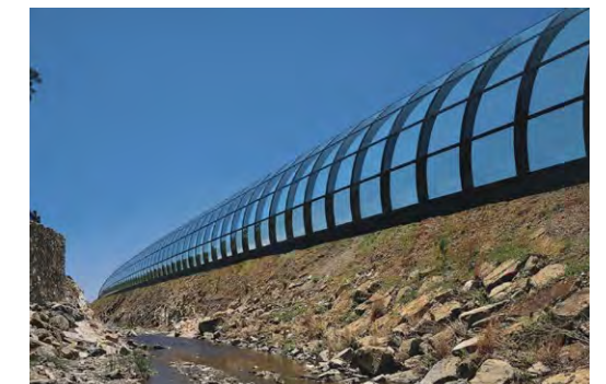
FIGURE 102 Demonstrates: semi-enclosed transparent noise wall to reduce visual bulk and allow light into the adjacent creek. Eastern Freeway, Melbourne. Design: Wood Marsh
