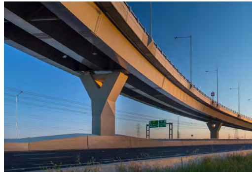
FIGURE 90 Refer Objective 3.2. Demonstrates: well considered multi span steel trough bridge with articulated piers and integral crosshead. M80 Ring Road, Melbourne. Design: Peter Elliott and VicRoads, Photography: John Gollings
