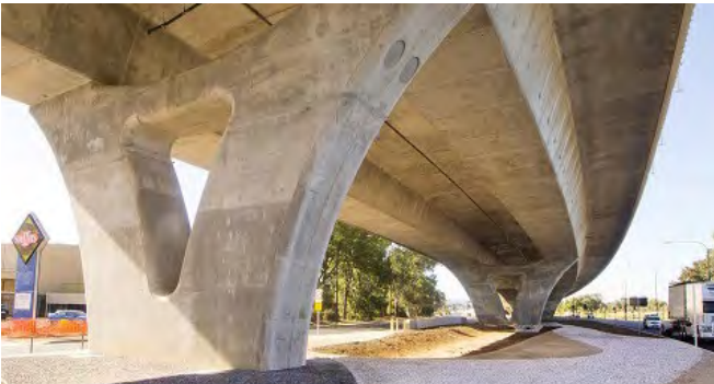
FIGURE 1 Demonstrates: well considered pier forms integrated with super structure, providing clear visual permeability across the ground plane. South Road Superway, Adelaide. Design: Wood Marsh, Image: GHD
