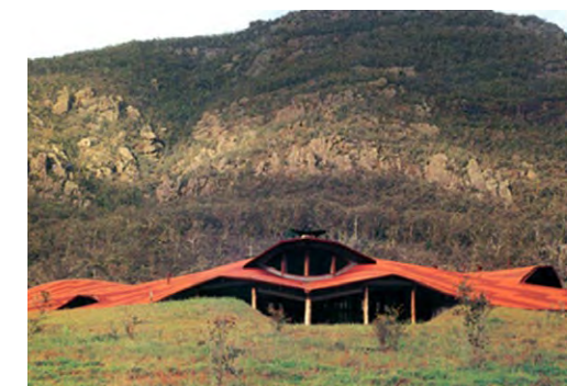
FIGURE 129 Refer Objective 1.1. Demonstrates: context sensitive design reflecting cultural values. Brambuk Cultural Centre, Halls Gap VIC. Architect: Gregory Burgess Architects Photography: Trevor Mein
