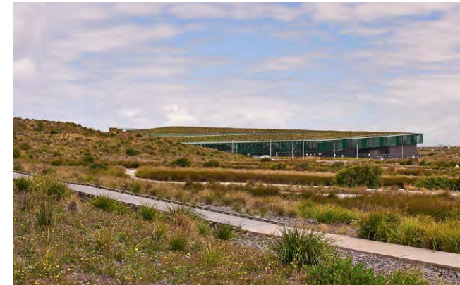
FIGURE 24 Demonstrates: green roof which integrates building with surrounding landscape. Victorian Desalination Plant, Victoria. Design: ASPECT Studios, Photography: Peter Bennetts
