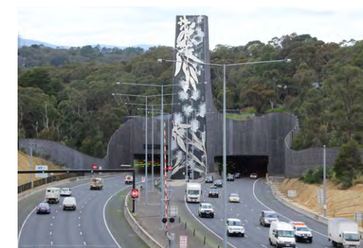
FIGURE 118 Refer Objective 1.5. Demonstrates: creative response and landmark feature that celebrates local context. Mullum Mullum Tunnel, EastLink, Melbourne. Design: Wood Marsh and Tract Consultants, Image: VicRoads
