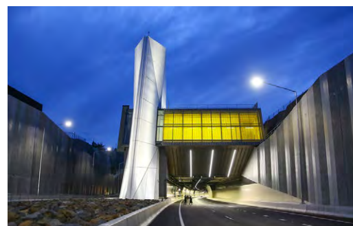
FIGURE 151 Refer Objective 1.5. Demonstrates: integrated ventilation structure and tunnel approach. Waterview Tunnel, Auckland. Design: Warren and Mahoney, Image: NZ Transport Agency
