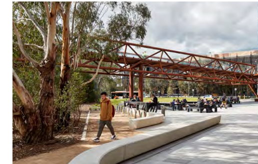
FIGURE 143 Demonstrates: well utilised public open space beneath pedestrian bridge at university campus. Burwood Link Bridge, Melbourne. Design: Watson Architecture and GHD, Image: GHD
