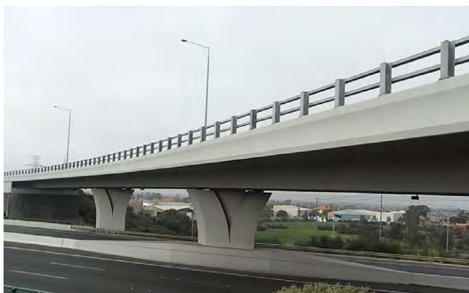
FIGURE 9 Demonstrates: a well designed substructure, integrated pier / details and appropriate integration of safety barriers. Western Ring Road, Hume. Image: VicRoads
