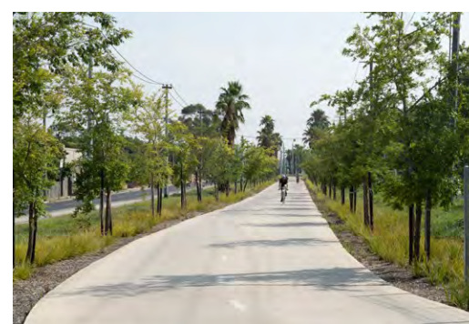
FIGURE 110 Demonstrates: good quality planting along water easement. St Georges Road, Thornbury. Image: NELP
