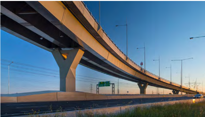
FIGURE 2 Demonstrates: well considered multi span steel trough bridge with articulated piers and integral crosshead. M80 Ring Road, Melbourne. Design: Peter Elliott and VicRoads, Photography: John Gollings
