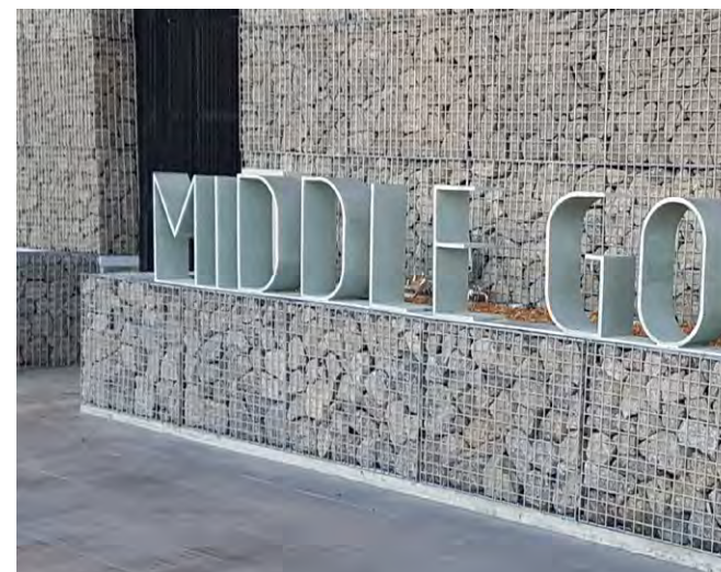
FIGURE 88 Demonstrates: reuse of reclaimed site materials in project design. Middle Gorge Station as part of the South Morang line to Mernda extension. Design: Grimshaw, Image: NELP
