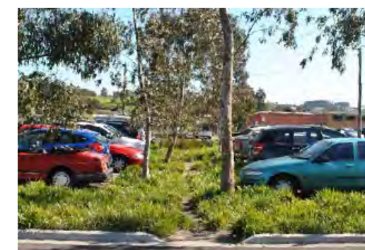
FIGURE 106 Demonstrates: Water Sensitive Urban Design infrastructure and tree planting incorporated into the car park. Henry Turner Oval car park, Melbourne. Design: GHD
