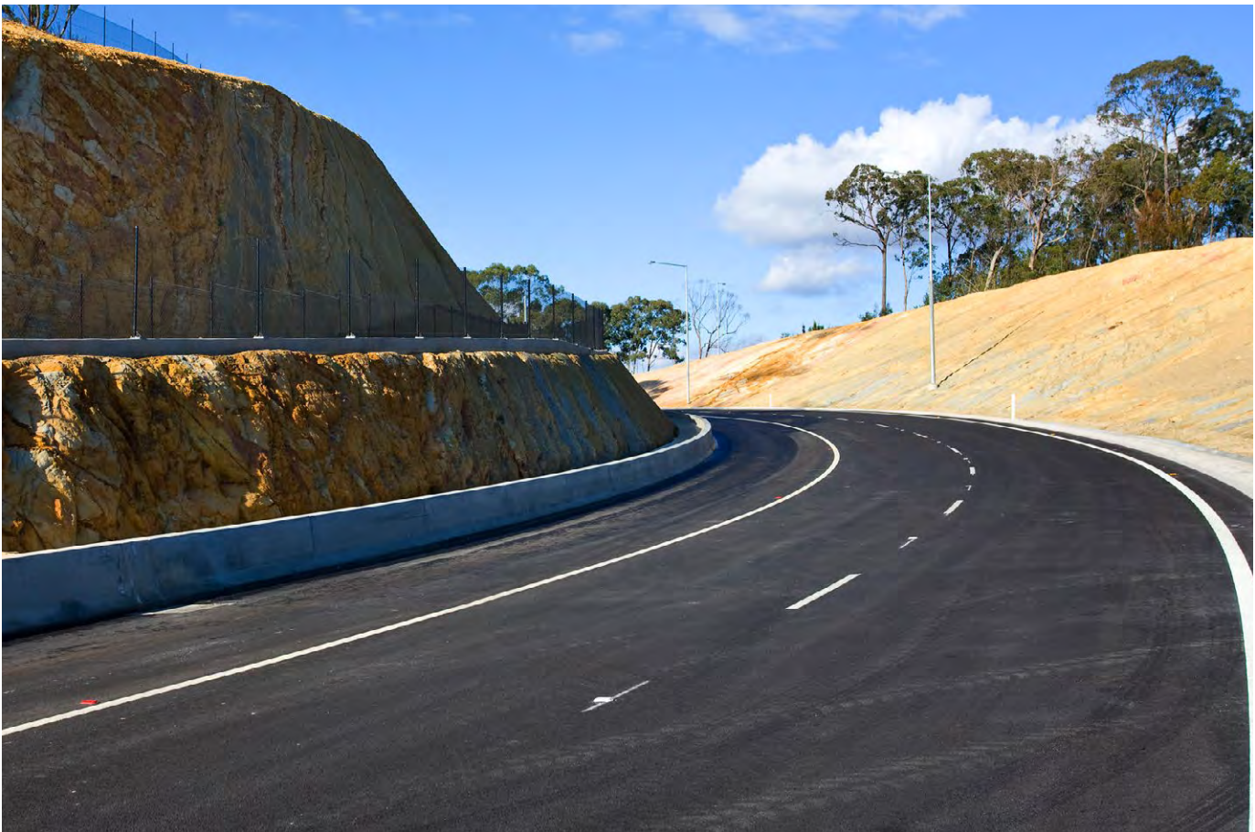
FIGURE 16 Demonstrates: use of existing natural stone in cutting as a design feature. EastLink Freeway, Melbourne. Design: Wood Marsh and Tract Consultants, Image: EastLink
