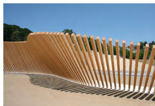
FIGURE 130 Demonstrates: dynamic and sculptural screening near tunnel entrance. Veduggio-Cassarate Tunnel Development, Switzerland. Design: Cino Zucchi Architetti
