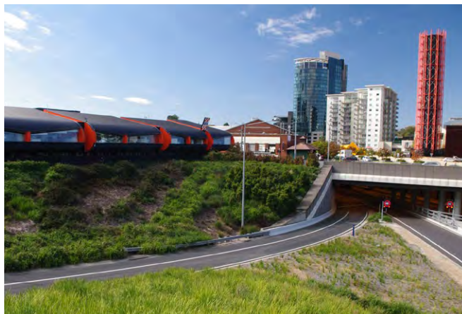
FIGURE 18 Demonstrates: well integrated tunnel approach which minimises impacts to surroundings. CityLink Western Tunnel portal, Melbourne. Image: VicRoads
