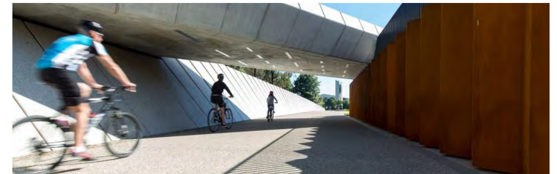
FIGURE 97 Demonstrates: use of natural light and a generous proportioned underpass. Bowen Place Crossing, Canberra Design: Lahz Nimmo Pty Ltd and Spackman Mossop Michaels, Photography: Brett Boardman
