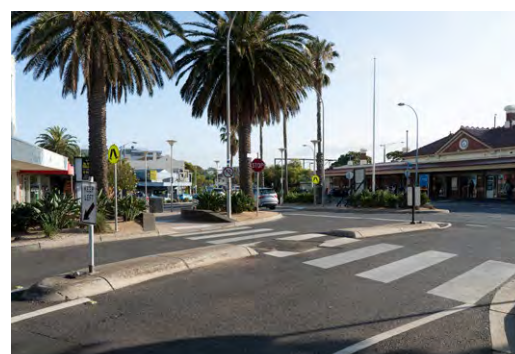
FIGURE 103 Refer Objective 3.1. Demonstrates: connectivity of train station to town centre and surrounds. Sandringham Village, Victoria. Image: NELP
