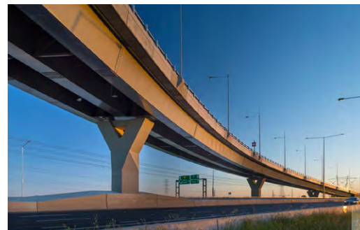
FIGURE 145 Refer Objective 3.2. Demonstrates: well considered multi span steel trough bridge with articulated piers and integral crosshead. M80 Ring Road, Melbourne. Design: Peter Elliott and VicRoads, Photography: John Gollings
