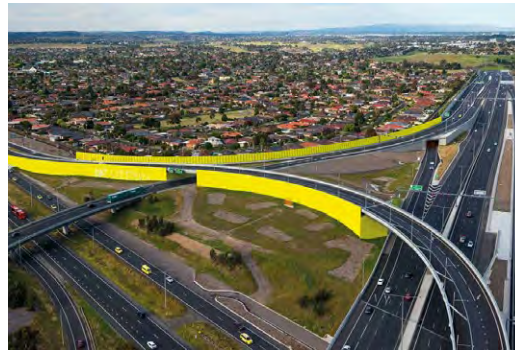
FIGURE 89 Refer key place-specific requirement 3A. Demonstrates: an interchange celebrated as a gateway which assists with navigation in a complex interchange. M80, Melbourne. Design: Peter Elliott and VicRoads, Photography: John Gollings
