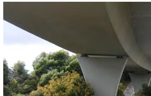
FIGURE 146 Refer Objective 3.2. Demonstrates: Planting that enhances visual amenity and softens built elements. Western Freeway, Warrenheip. Image: VicRoads
