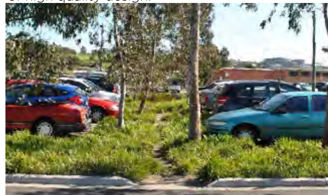
FIGURE 50 Demonstrates: Water Sensitive Urban Design infrastructure and tree planting incorporated into the car park. Henry Turner Oval car park, Melbourne. Design: GHD
