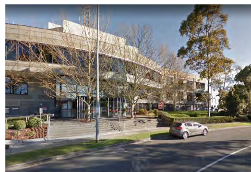
FIGURE 126 Refer Objective 3.3. Demonstrates: high quality commercial development with well vegetated frontage which could be enabled. Burwood, Melbourne. Image: Google
