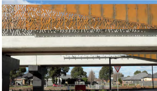
FIGURE 40 Demonstrates: privacy screens on bridge used to minimise overlooking to residential areas. Hawkstowe Station, Melbourne. Design: Grimshaw, Image: GHD
