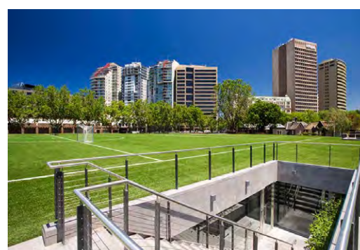
FIGURE 109 Demonstrates: integrated car park entry. Steele Oval underground car park at Melbourne Grammar, Melbourne. Design: Peter Elliott Architecture + Urban Design. Image: Peter Elliott
