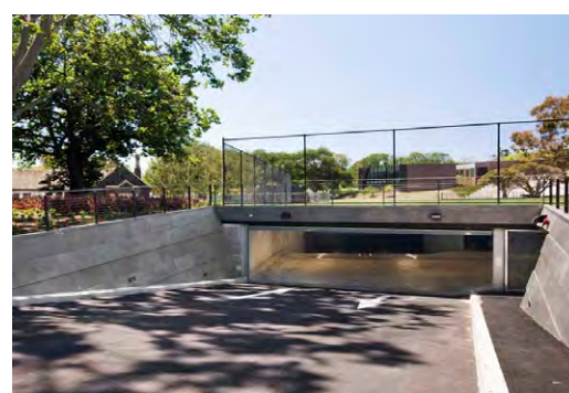
FIGURE 108 Demonstrates: integrated car park entry. Steele Oval underground car park at Melbourne Grammar, Melbourne. Design: Peter Elliott Architecture + Urban Design. Image: Peter Elliott
