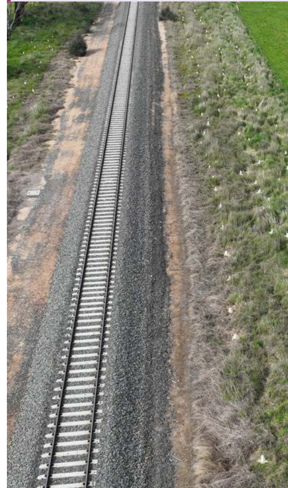
An aerial view of the recycled ballast located along the Shepparton Line – Photo by SCU Alliance
