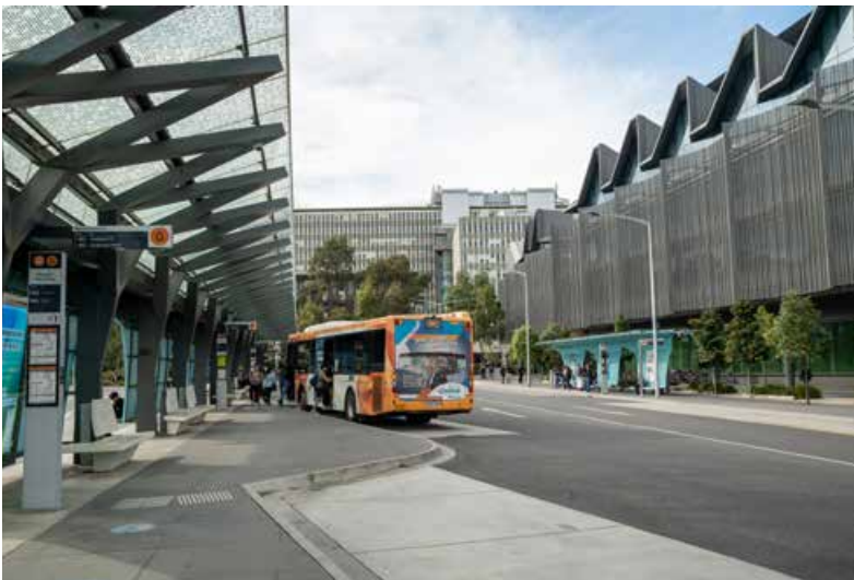
Monash University bus interchange
