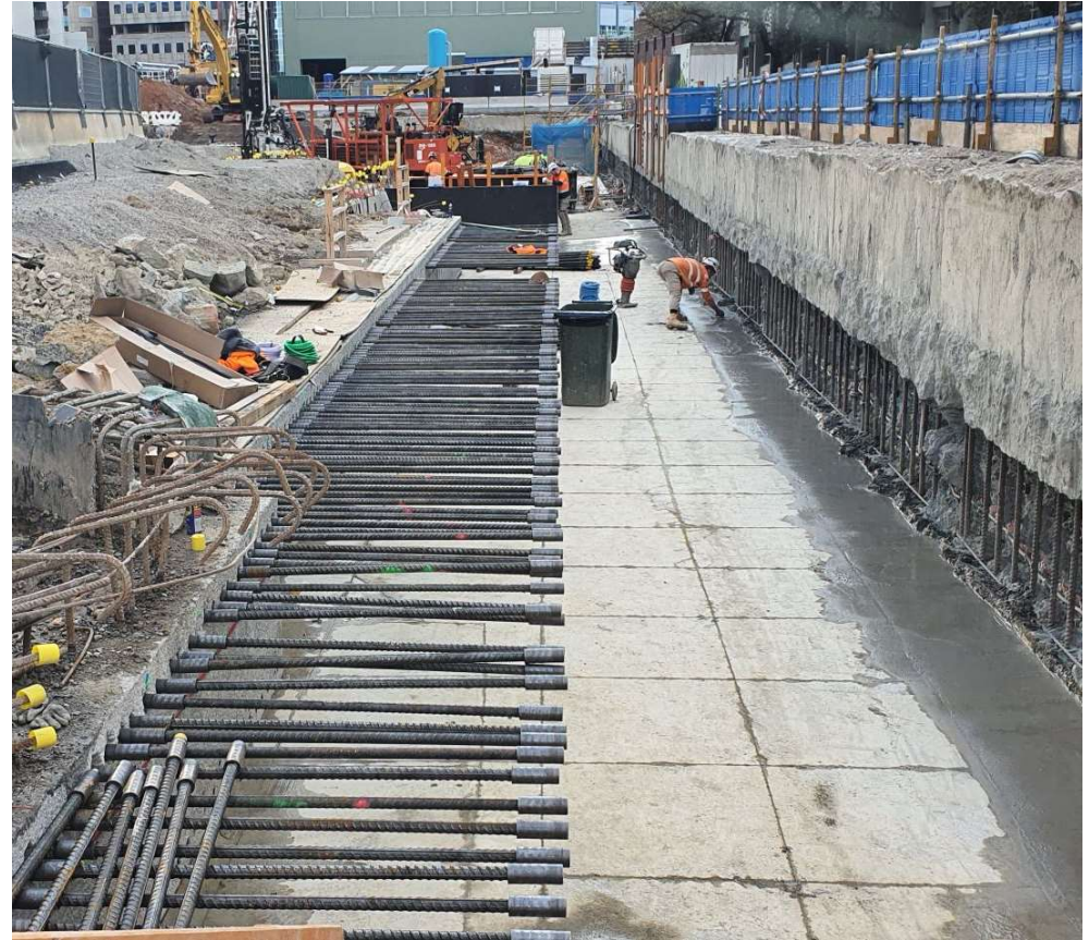
Installation of steel reinforcements
