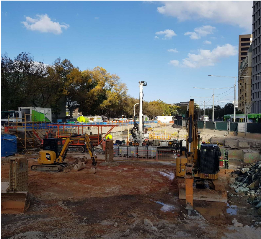
Excavation to roof slab level
