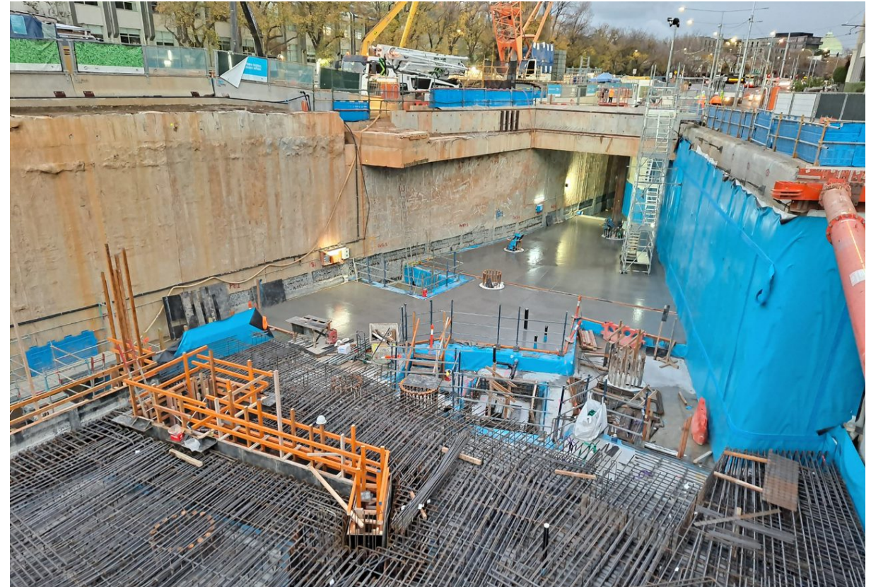
Tram Box Progress
