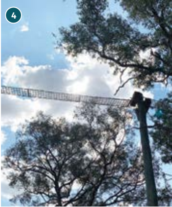
PROVIDE APPROPRIATE FAUNA CROSSINGS - ROPE BRIDGE, YAN YEAN ROAD UPGRADE STAGE 1
