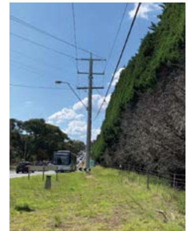
FIGURE 2.6: TYPICAL EXISTING ELECTRICITY TRANSMISSION LINE ALONG YAN YEAN ROAD CORRIDOR
