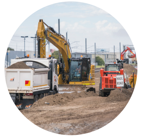
We've started major works on the new pedestrian and cyclist underpass.
