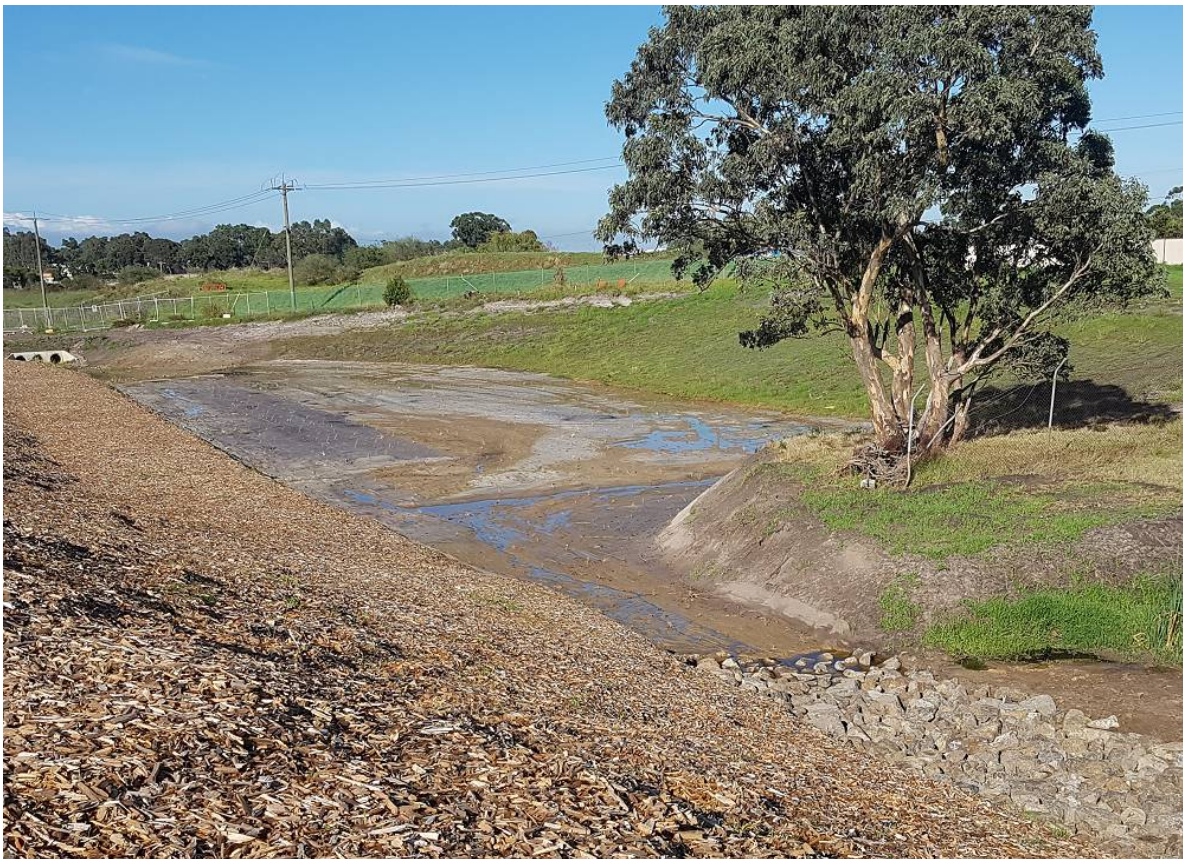
Above: Completed catchment pond in Area 1 with rock stabilised inlet channel (bottom right) and geofabric covered base which has been planted out with native grass.
