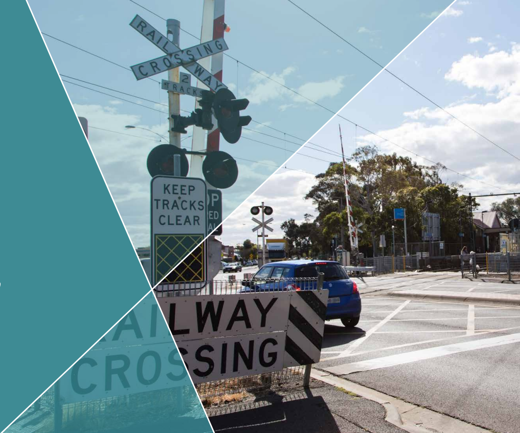
Current level crossing at Ferguson Street
