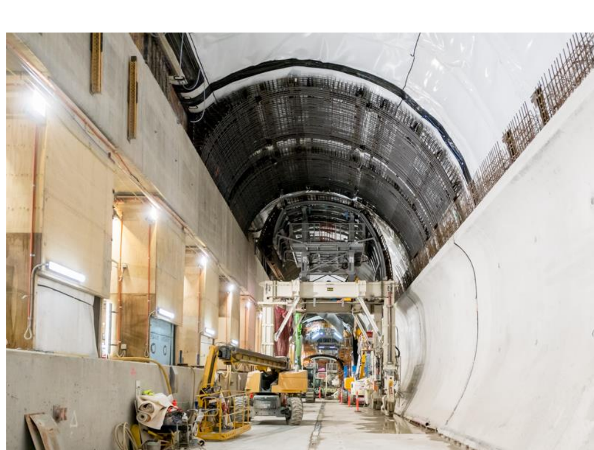
Arch reinforcement using a multi-purpose gantry
