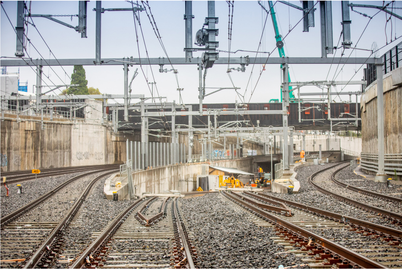
Newly installed rail tracks
