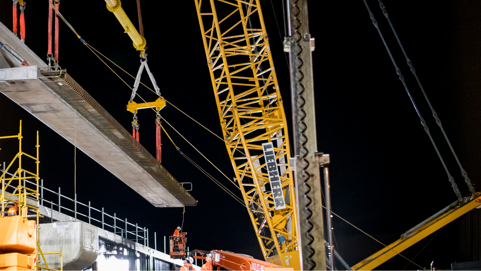
L-beam installation on the Reservoir Level Crossing Removal Project
