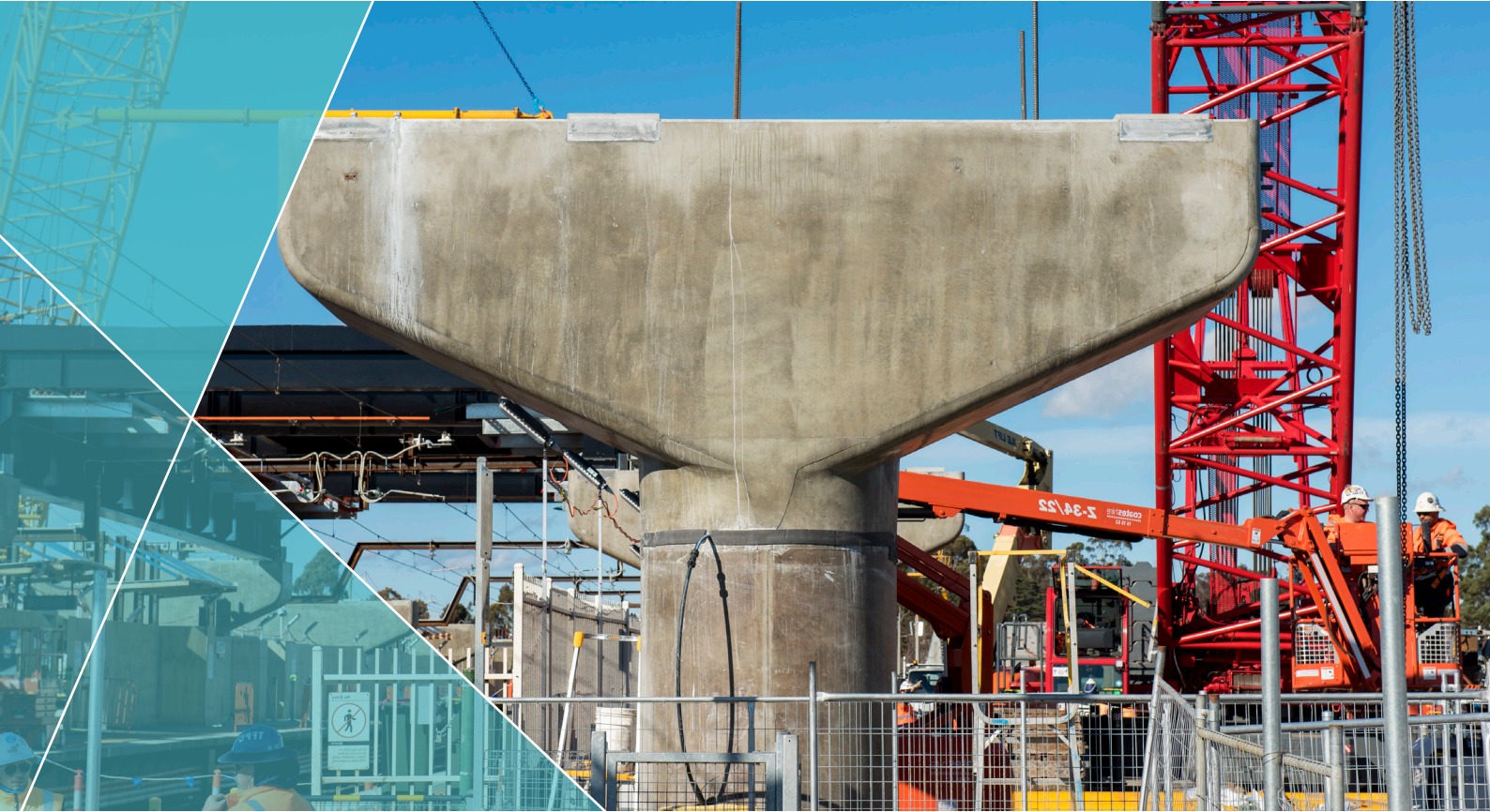
Pier and headstock installation during construction at the Reservoir Level Crossing Removal Project
