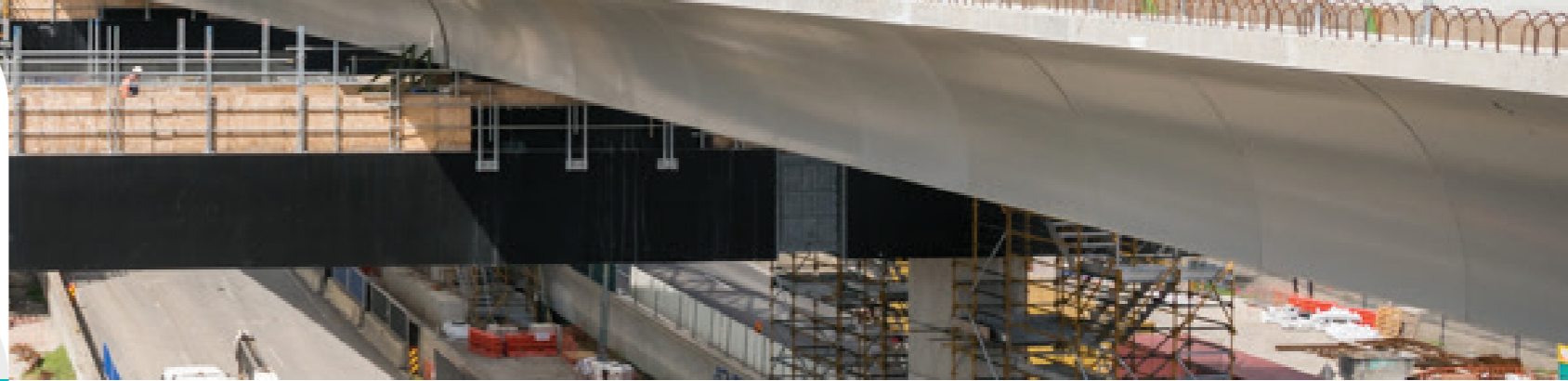
Elevated road construction on Footscray Road
