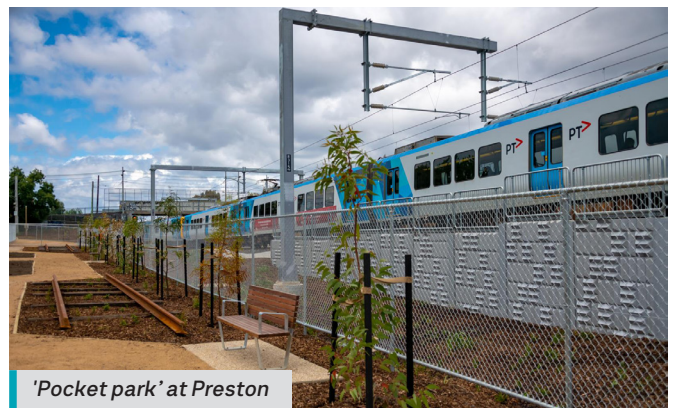
Salvaged railway sleepers and reused tracks
