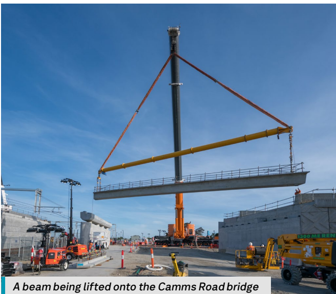
Our team connecting the beams to the road bridge
