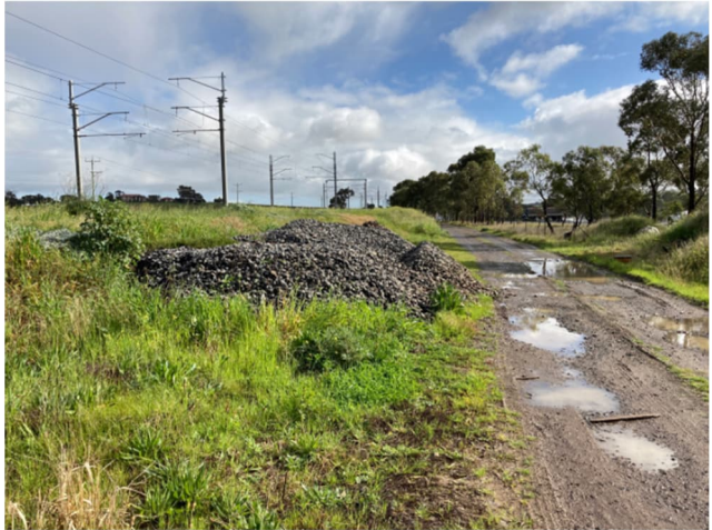
Plate 2 Material stock piling in the rail corridor
