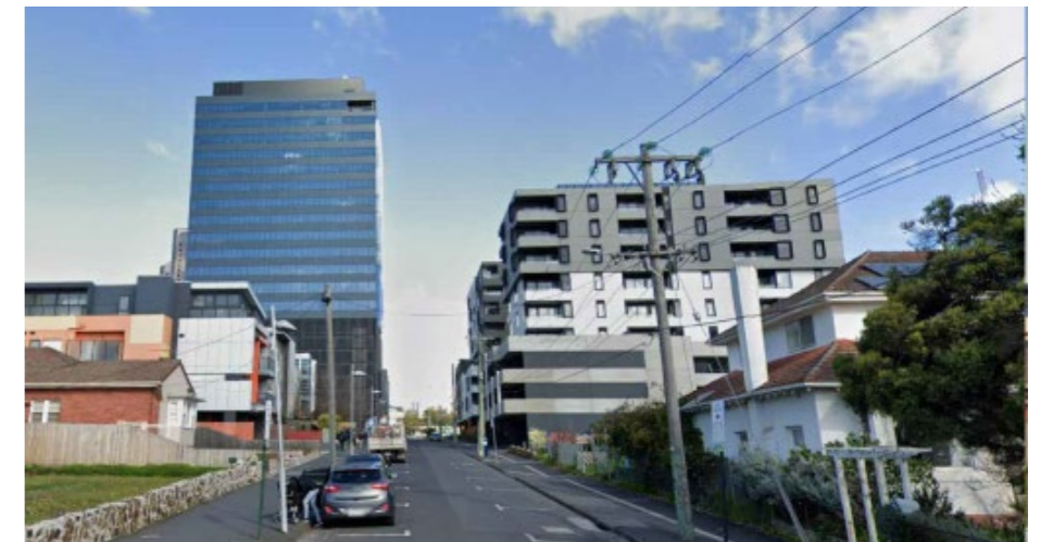
Figure A1.35: Box Hill Gardens looking southwards towards Bruce Street
