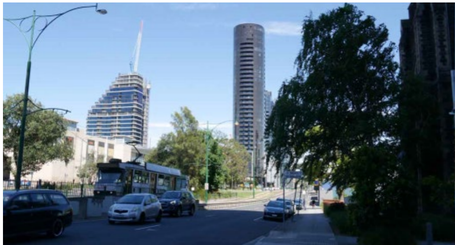
Figure A1.18: Widened Whitehorse Road
