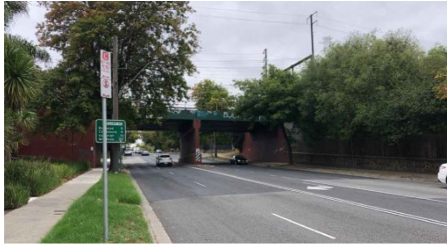
Figure A1.9: Vehicle and pedestrian underpass, Elgar Road.
