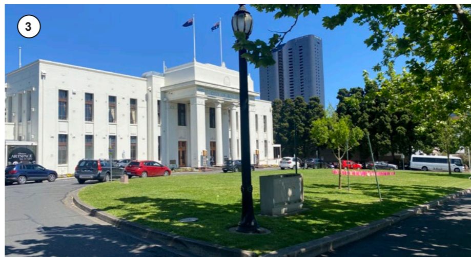
Figure B1.6: Box Hill Town Hall
