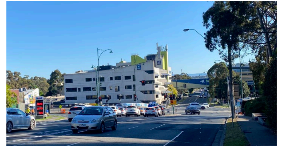
Figure A1.27: Elgar Road - north of the rail overpass
