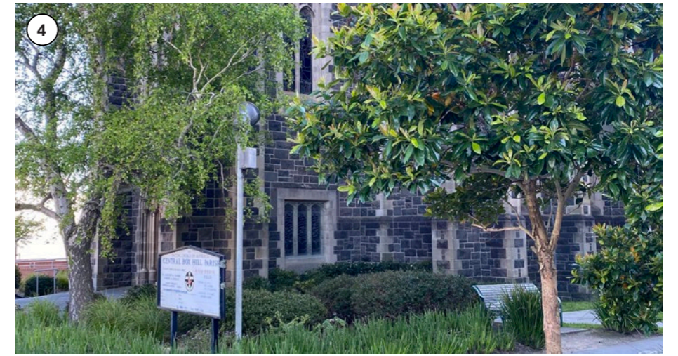
Figure B1.7: St Andrews Uniting Church
