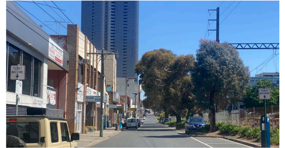
Figure A1.12: Interface with Railway Line, Rutland Road
