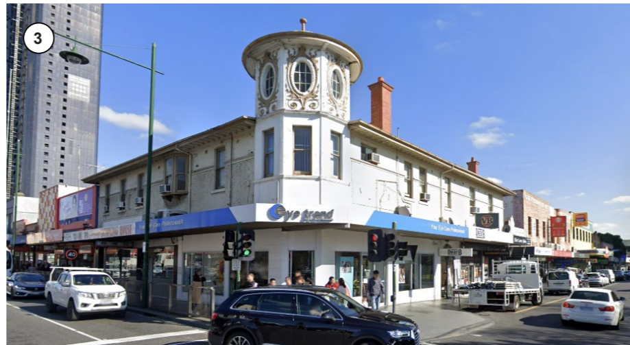
Figure B1.5: Former Railway Hotel
