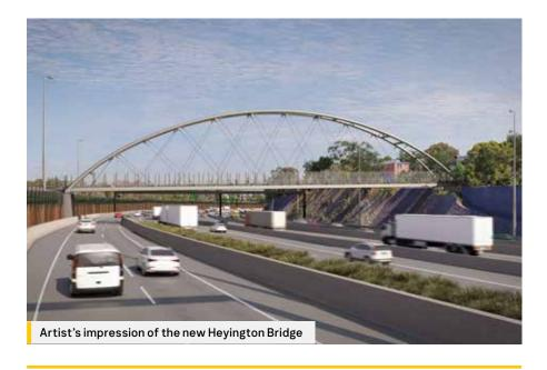
We'll remove some noise wall panels, install small piles, excavate and pour concrete to form the new northern bridge abutment - the structure at the end of the bridge that supports the bridge span.
