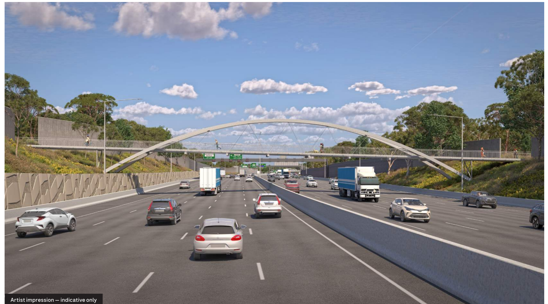
Figure 30: Retained bridge at Koonung Road upgraded for better pedestrian and cycling connectivity
