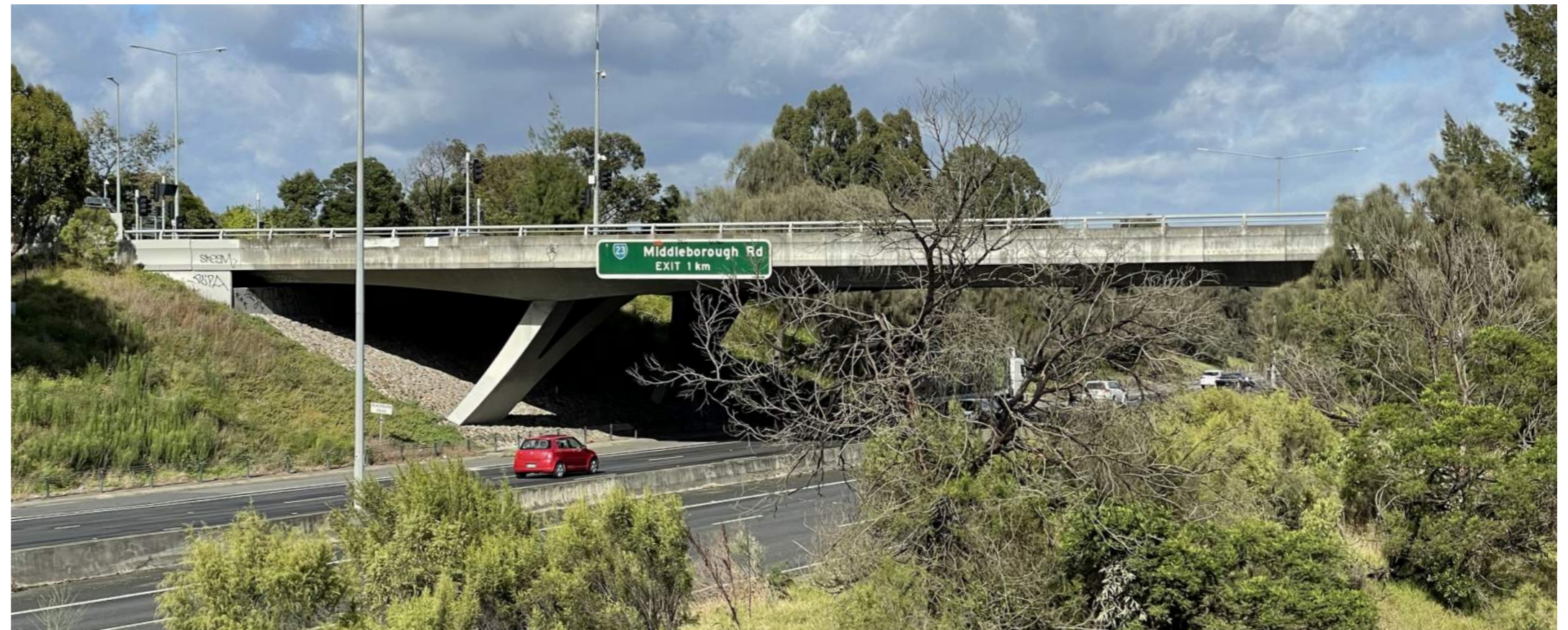
Figure 2: Eastern Freeway at Middleborough Road
