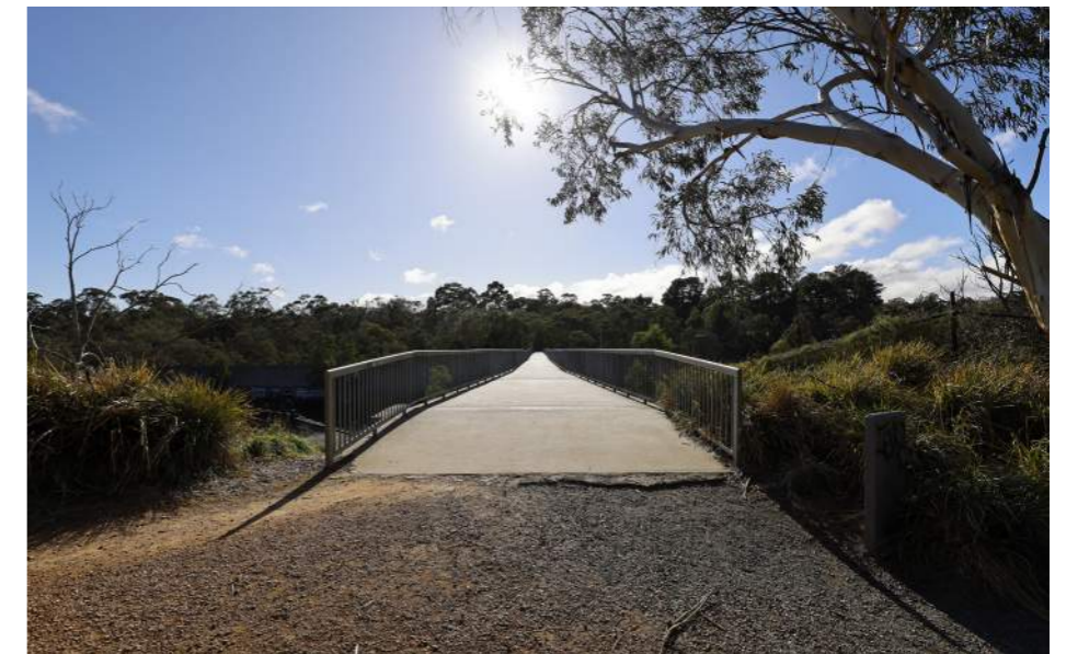
Figure 5: Existing Cabena Street pedestrian and cycling bridge approach
