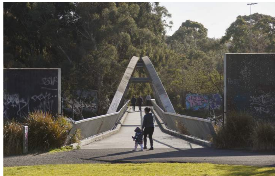
Figure 4: Existing Koonung Road pedestrian and cycling bridge approach
