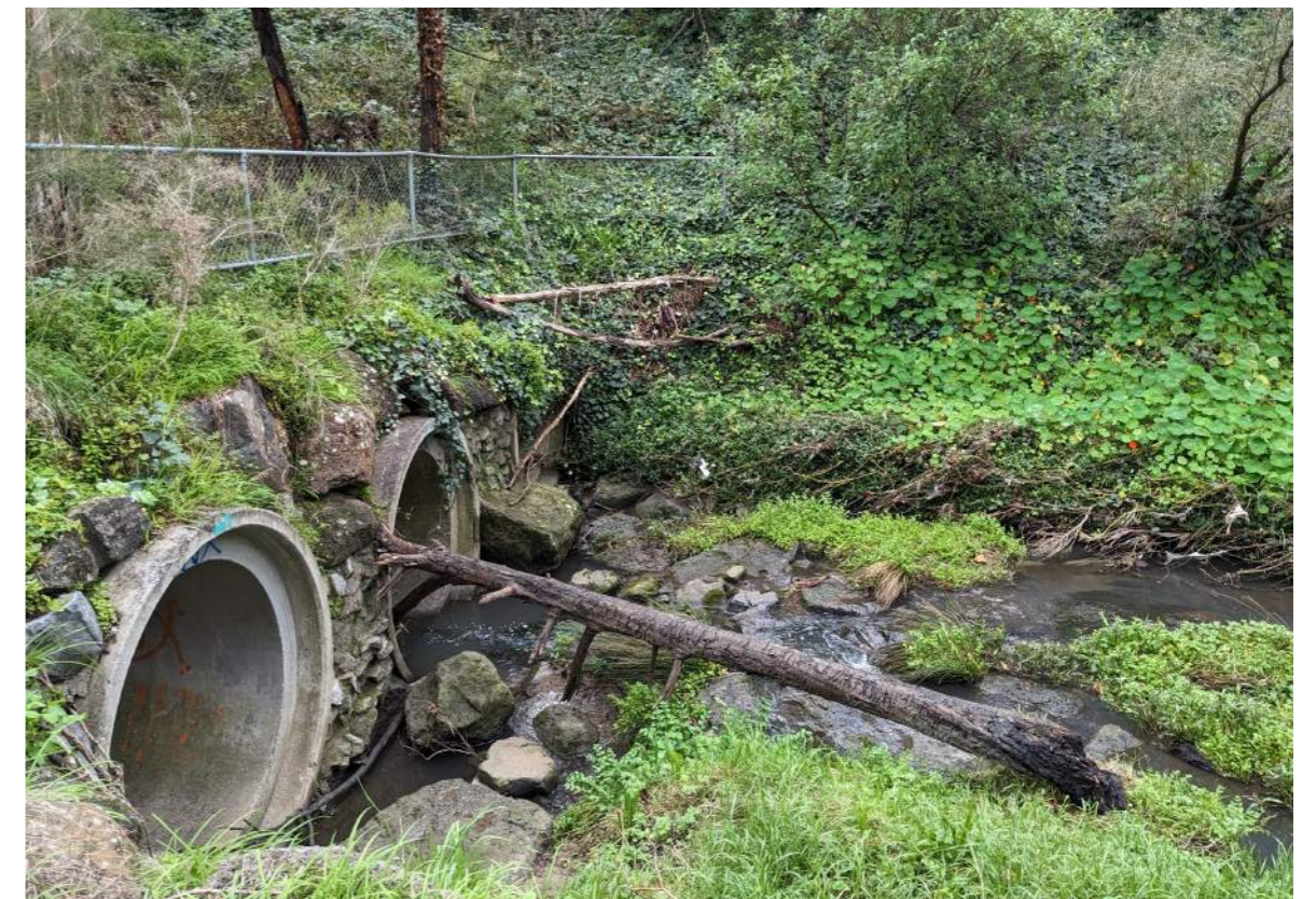
Figure 48: Koonung Koonung interface and culvert
