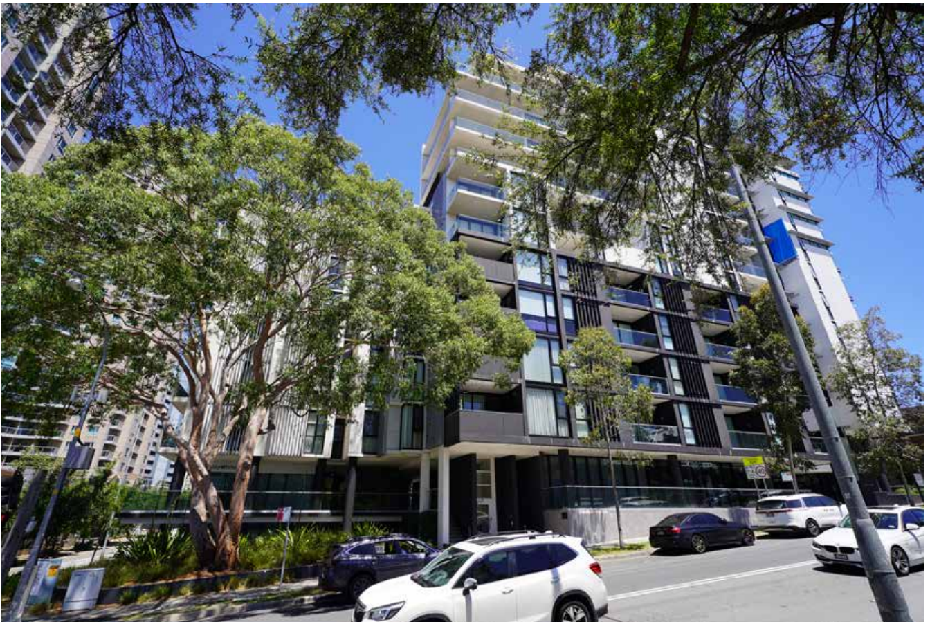
Mid-rise apartment developments, Sydney NSW
