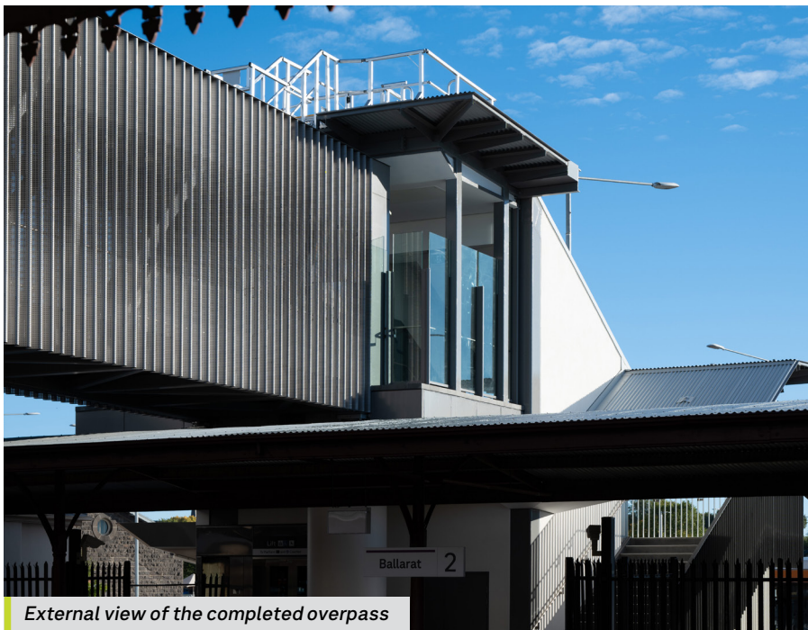
The new pedestrian overpass, lifted into place in November 2025
