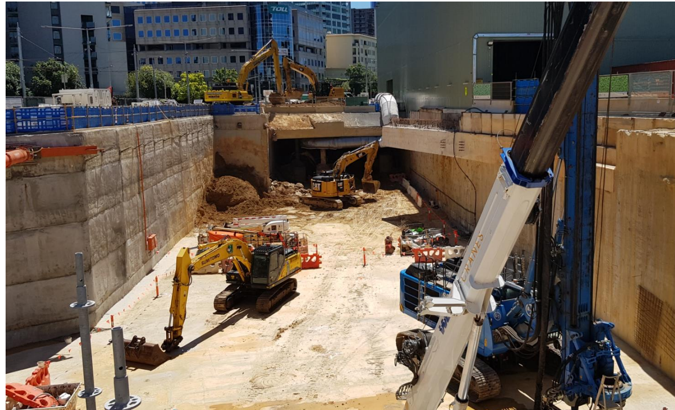
Piling has begun as excavation continues under the suspended slab
