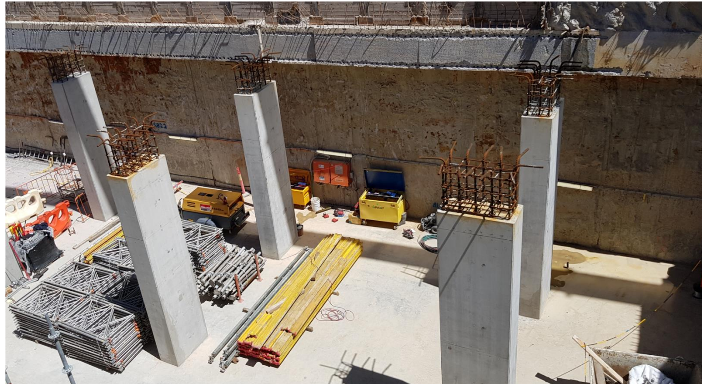
Internal columns poured in the Shrine entrance
