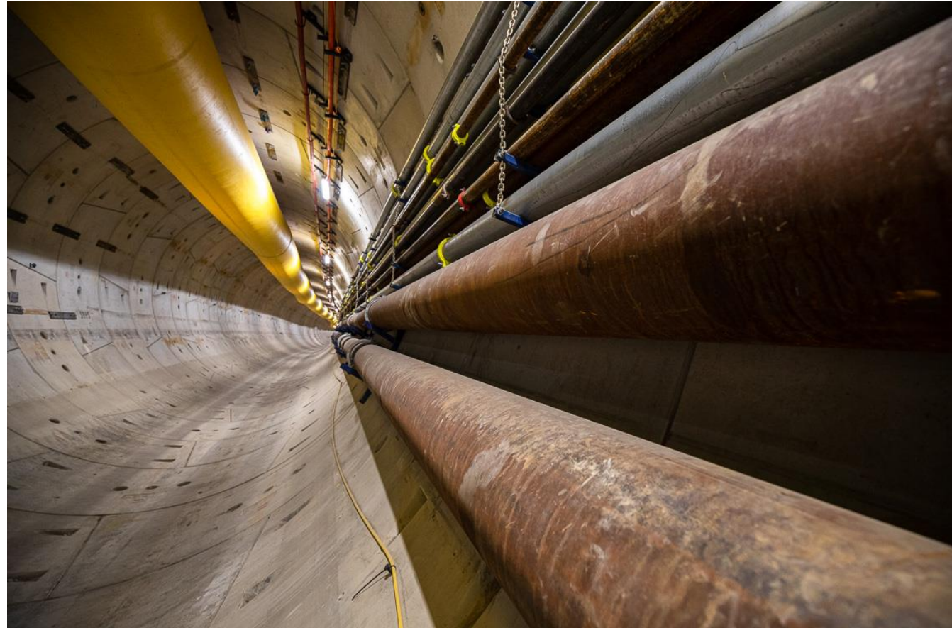
Pipes transporting excavated material
