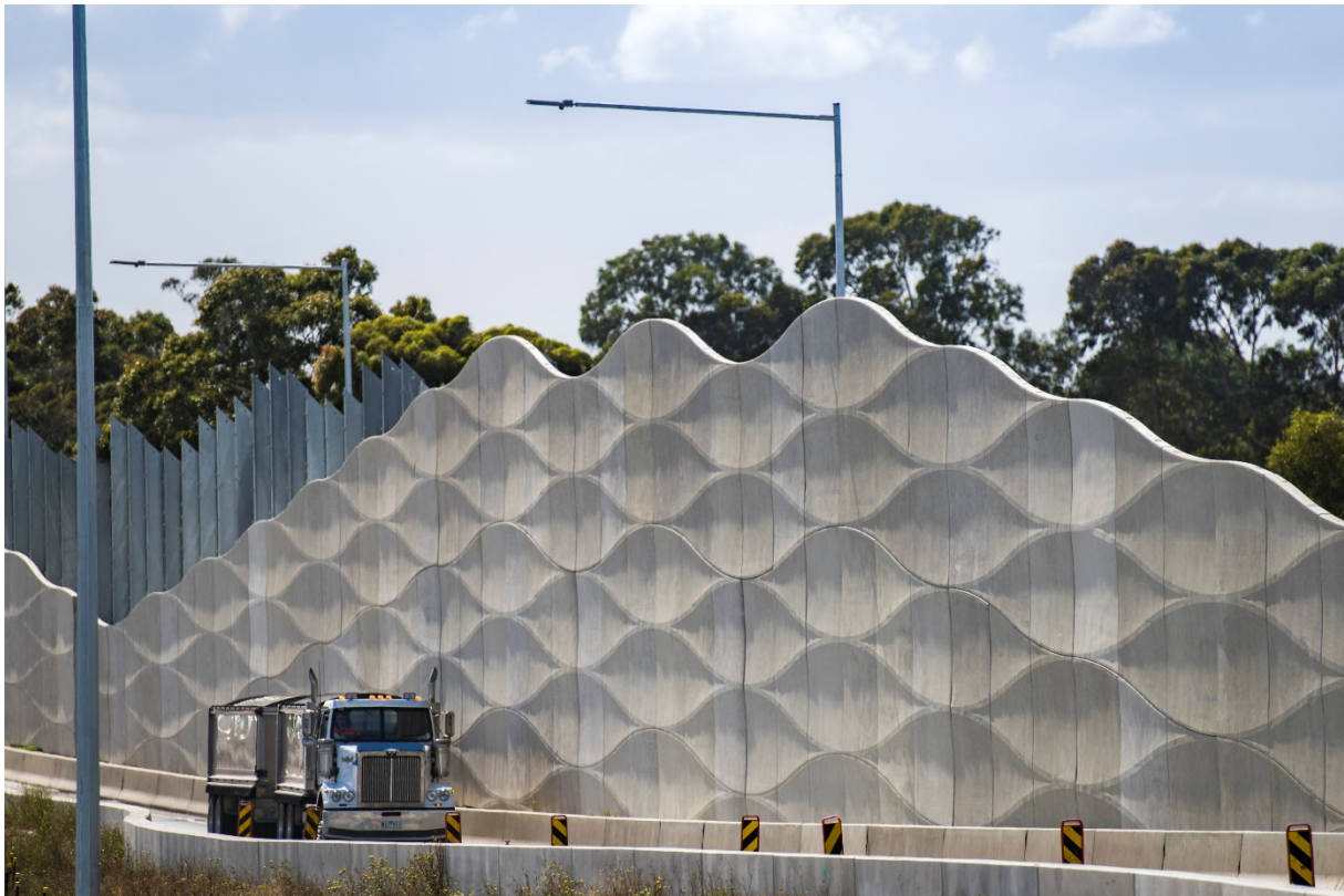
New noise walls installed along the Grieve Parade outbound exit ramp, Brooklyn
