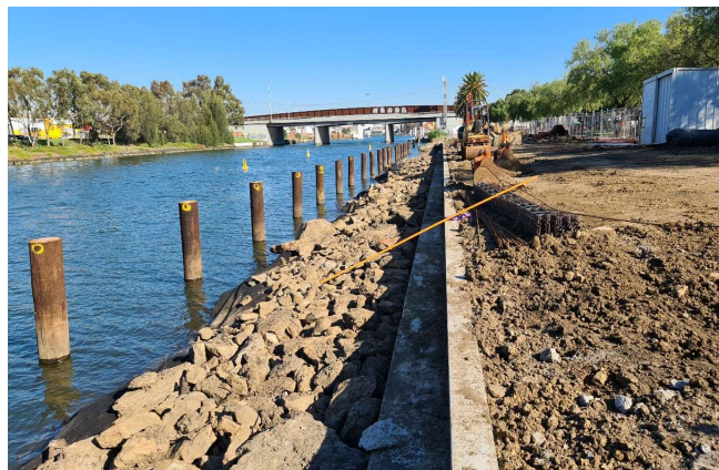
Rock beaching on the southern side of Bunbury Bridge
