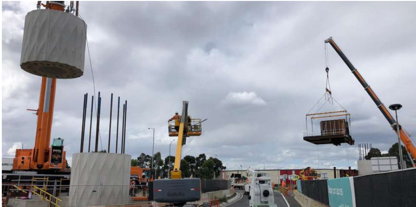
Column segments being installed at MacKenzie Road
