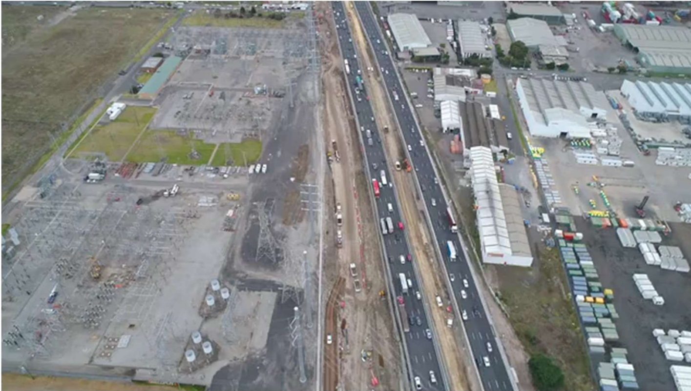
Drone footage of the Tunnel portals
