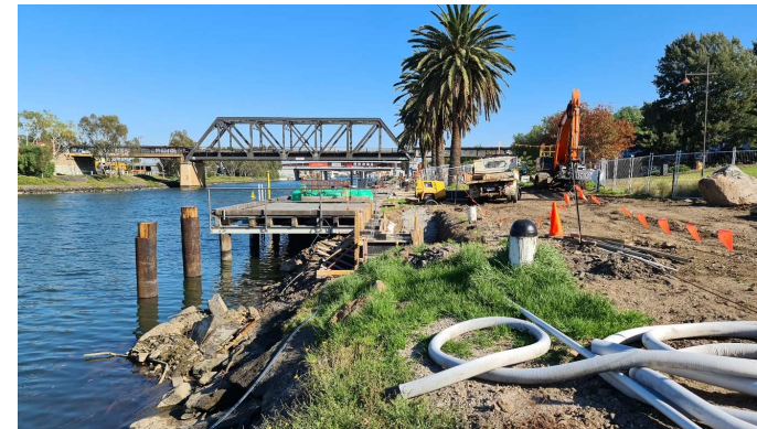
Northern side lower landing – abutment formwork
