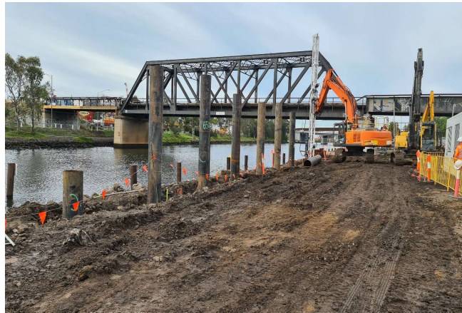
Steel piling on the northern side of Bunbury Bridge
