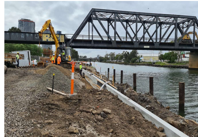
Compaction behind the abutment on the southern side of Bunbury Bridge
