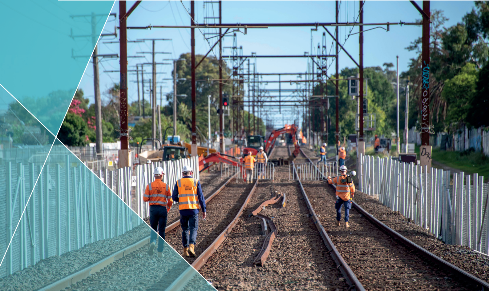
Construction underway on the Preston Level Crossing Removal Project.
