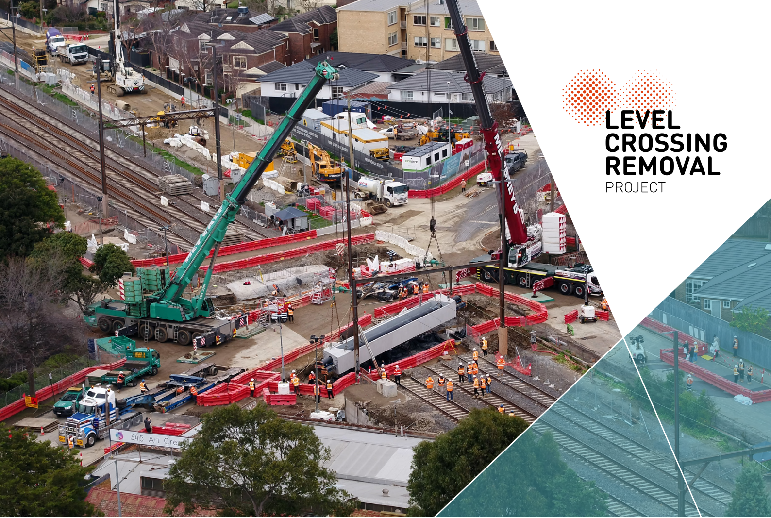
A beam being lifted into place on Mont Albert Road
