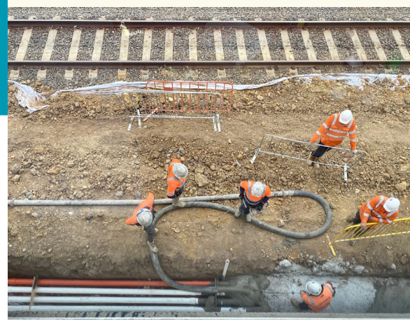
Relocation of communication cables along the rail line earlier this year
