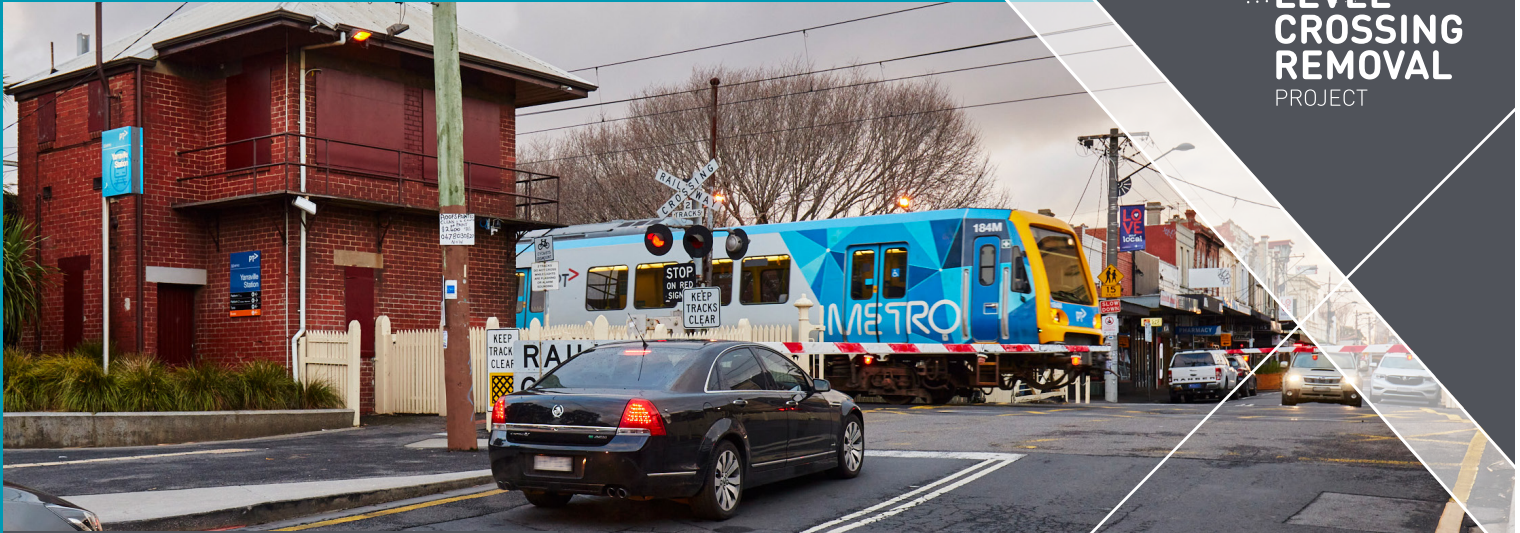
Level crossing at Anderson Street, Yarraville
