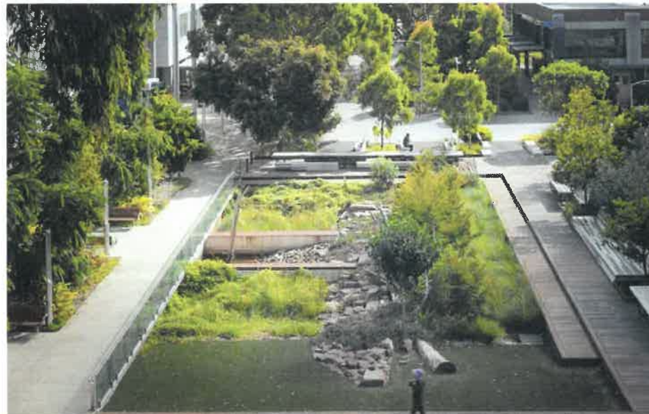
QB26 - Monash Biobasin, Monash Western Precinct, Clayton, VIC Demonstrates a well-integrated and compact stormwater harvesting system that captures, treats and stores stormwater for irrigation reuse. Design: Rush Wright Associates. Photographer: John Gollings.
