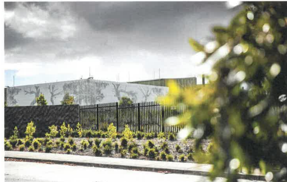
QB09 - Brunswick Power Terminal Station, Brunswick, VIC Demonstrates a well-designed site boundary treatment and a public realm interface that is comfortable and attractive for pedestrians. Design: Beca Pty Ltd. Photographer: Marcus Enno Photography.
