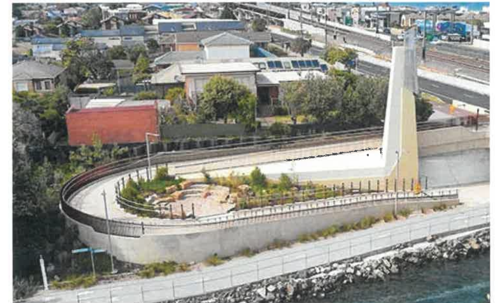
QB19 - Karrum Karrum Bridge, Carrum, VIC Demonstrates the sensitive integration and interpretation of indigenous themes at a key location within the movement network. Design: Rush Wright Associates, Photographer: Latitude Photography/Peter Clarke.
