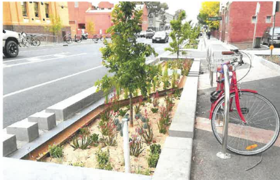
QB25 - Brunswick Town Hall, Brunswick, VIC Demonstrates well-integrated WSUD infrastructure and landscaping that is well-integrated with the streetscape. Design: Moreland City Council Image: Moreland City Council
