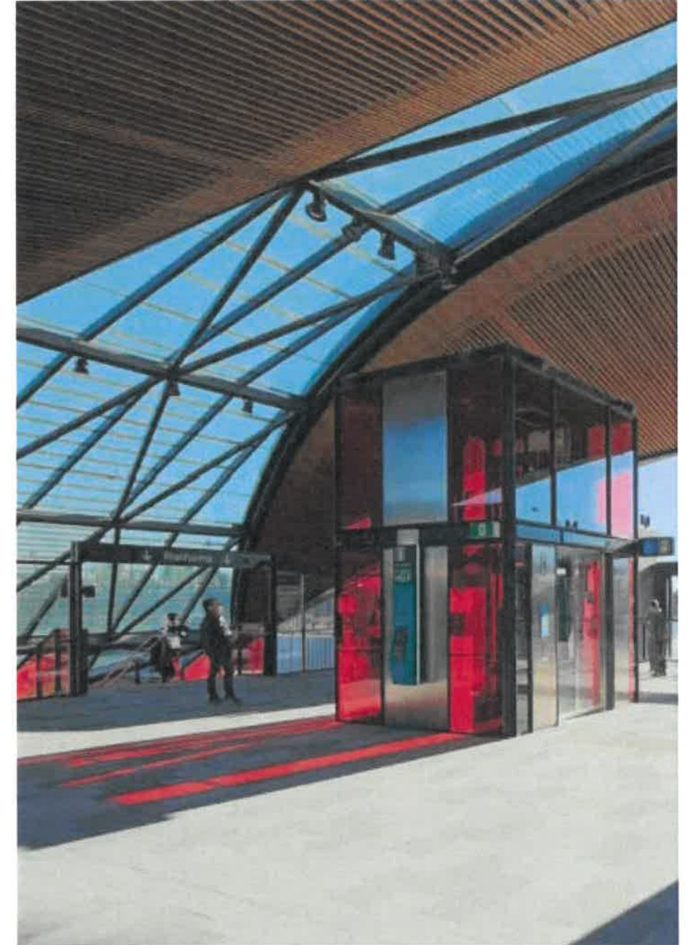
QB02 - Cherrybrook station, Metro North West, Cherrybrook, NSW Demonstrates a welcoming station entrance that is attractive and comfortable for users. Design: Hassell. Photographer: Ian Hobbs.
