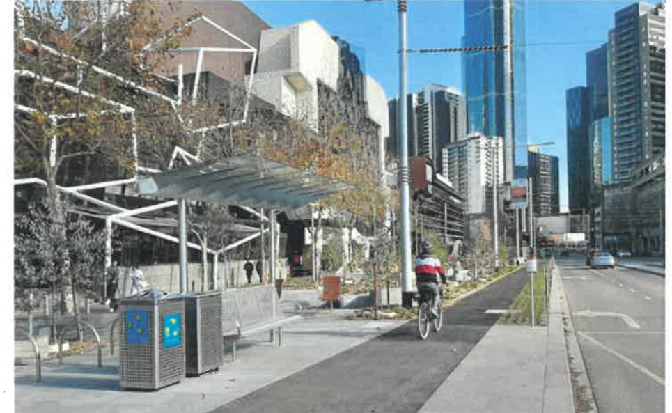
QB34 - Southbank Boulevard, Melbourne, VIC Demonstrates successful integration of cycle route into coherent streetscape design. Design: Melbourne City Council. Image: Augustus Brown.
