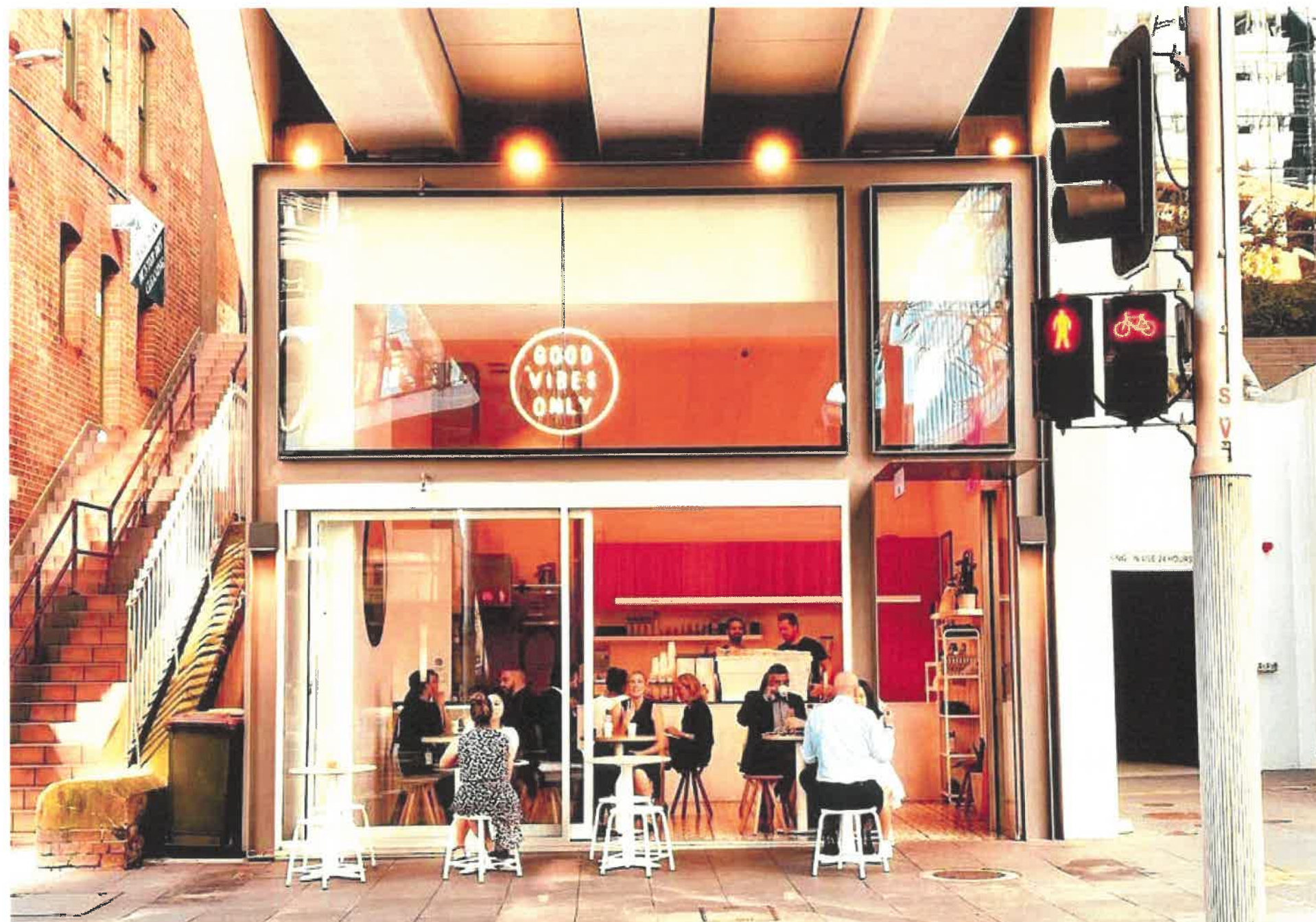
QB47 - Sussex Street pedestrian bridge, Sydney, NSW Demonstrates space below an elevated structure that enhances place outcomes and feelings of safety in the public realm. Design: Wood Bagot. Image: Good Vibes Only.
