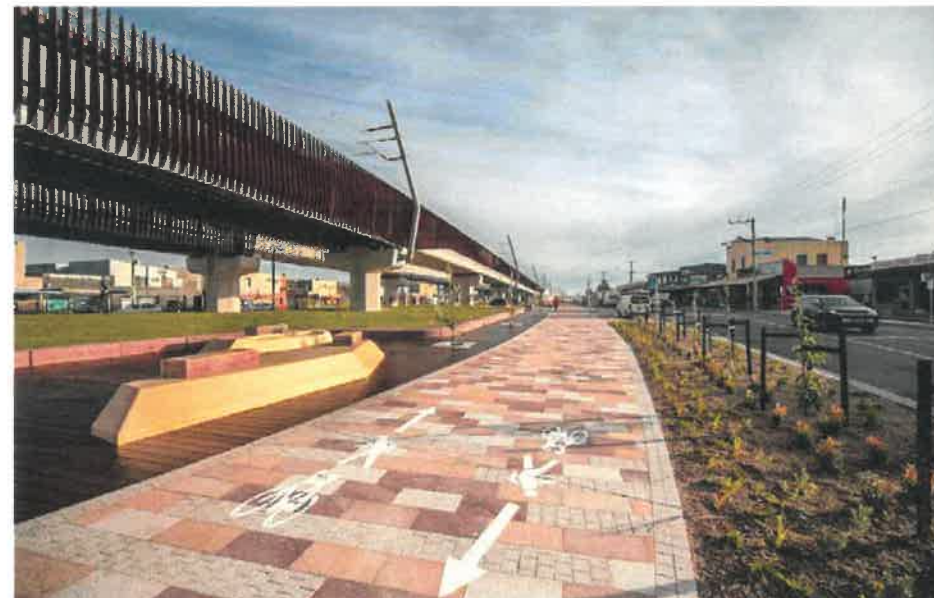
QB48 - Carrum station, VIC Demonstrates the use of public realm materials to define space allocation for different transport modes. Design: Rush Wright Associates. Image: Level Crossing Removal Project.
