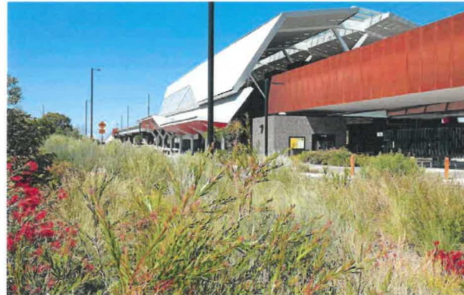
QB21 - Hawkstowe station, VIC Demonstrates locally responsive planting design that requires low maintenance. Design: Woods Bagot. Image: Level Crossing Removal Project.
