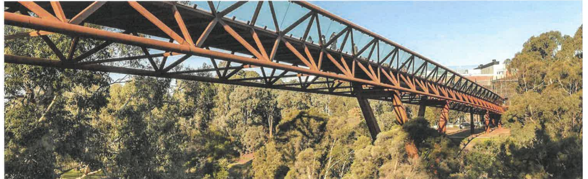
QB44 - Burwood Link, Burwood, VIC Demonstrates a structurally expressive bridge structure that is contextually sensitive. Design: watson architecture+design. Photographer: Lisbeth Grossmann.
