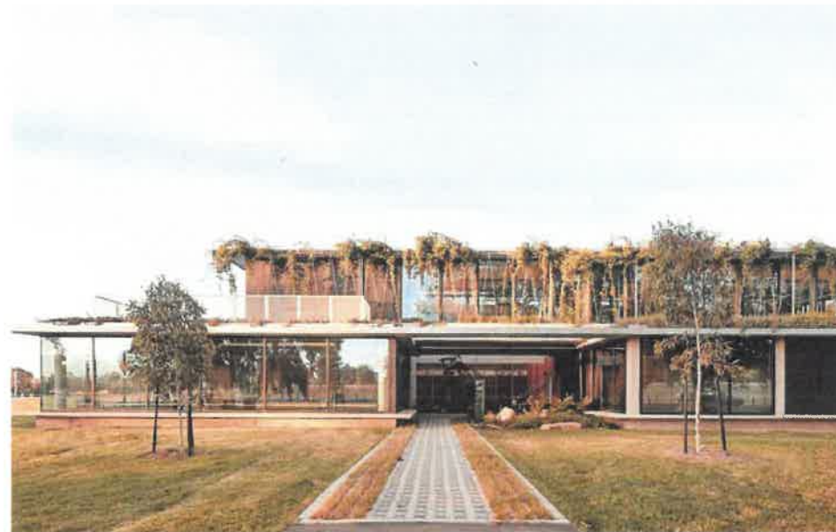
QB08 - Albert Park Office and Depot, Melbourne, VIC Demonstrates a well-designed building that sits comfortably in its context and contributes to positive place outcomes. Design: Archier, Harrison and White. Photographer: Peter Bennetts.
