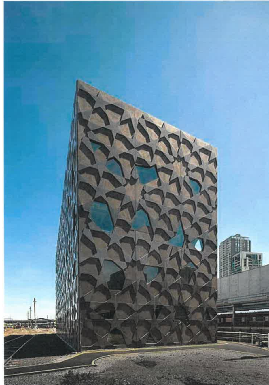
QB11 - The Yardmaster's Building, Southern Cross Station, Melbourne, VIC Demonstrates a visually interesting design that maintains a high quality treatment to views from all directions. Design: McBride Charles Ryan. Photographer: John Gollings.
