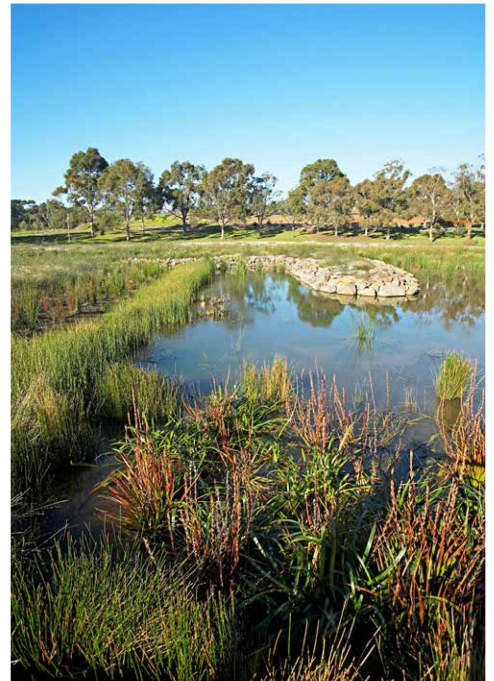
QB27 - Royal Park Wetland, Melbourne, VIC Demonstrates attractive stormwater harvesting and water quality treatment in a constructed wetland. Design: Rush Wright Associates. Photographer: Michael Wright
