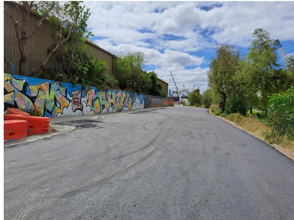
Lyons Street resurfacing
