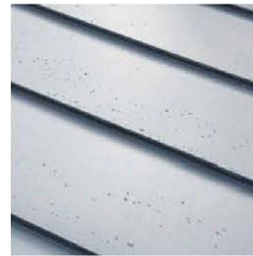
Metal Roof Covering Entry Portal & City Square Ancillary Structures
