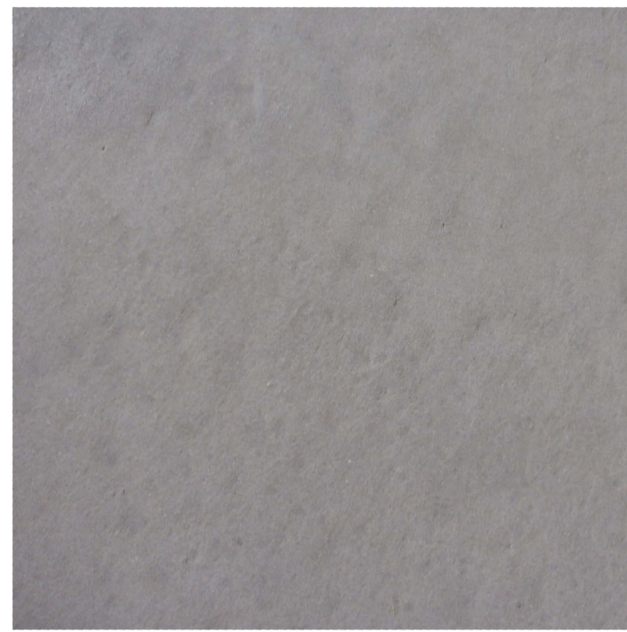
Insitu Concrete - Class 2
