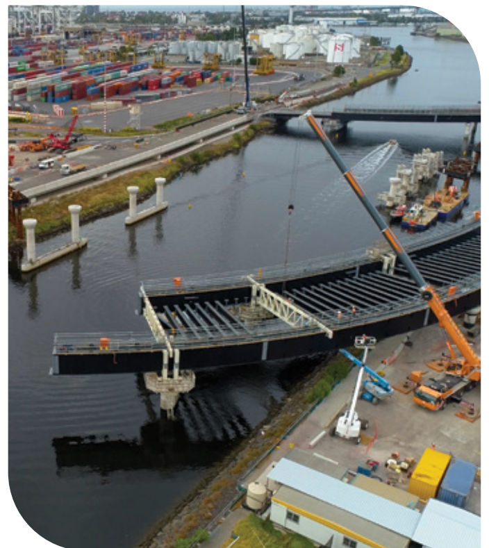
Steel beams for new Maribyrnong River bridges
