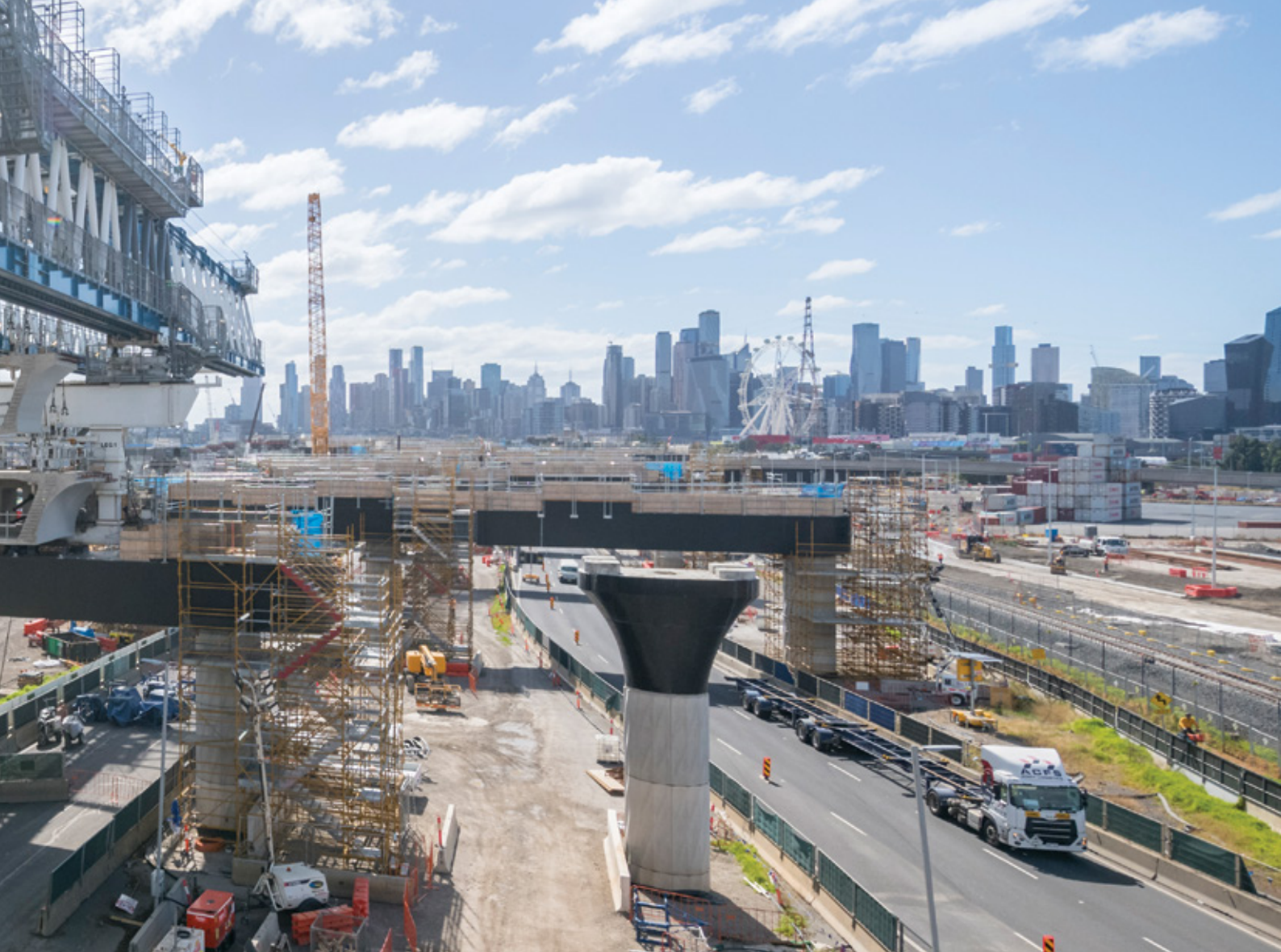
Elevated road construction on Footscray Road
