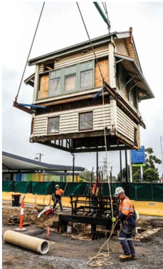
The signal box being lifted from its old site
