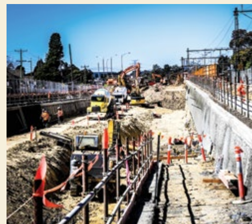
Construction of the lowered rail cutting alongside Ca
