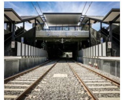
The new lowered rail line
