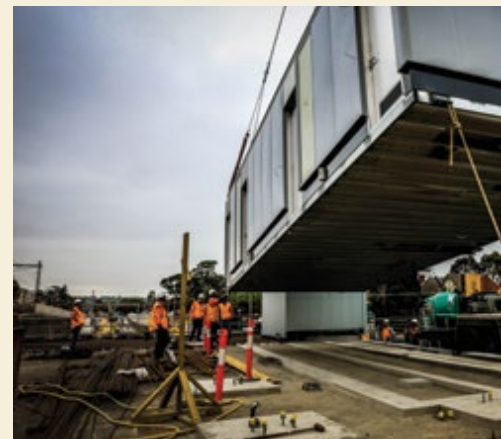
Lowering the pre-fabricated station building into pla
