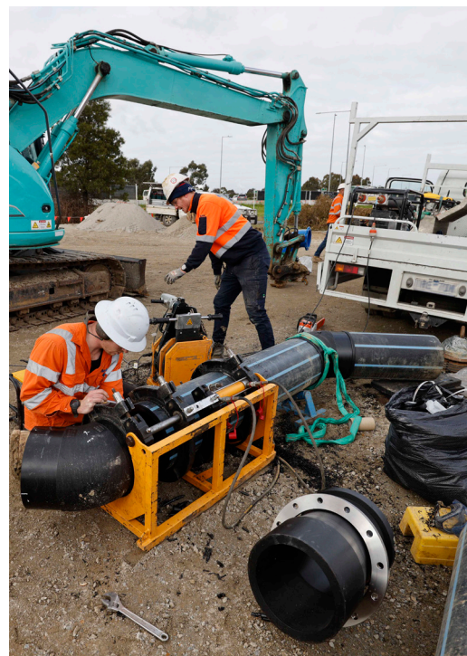
Above: Water utility relocation taking place on Healesville-Koo Wee Rup Road
