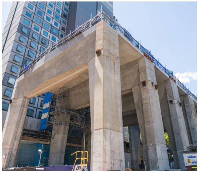
Main station entrance at Swanston and La Trobe Streets
