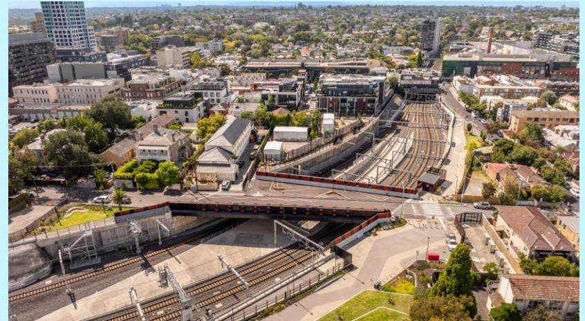
After – William Street bridge
