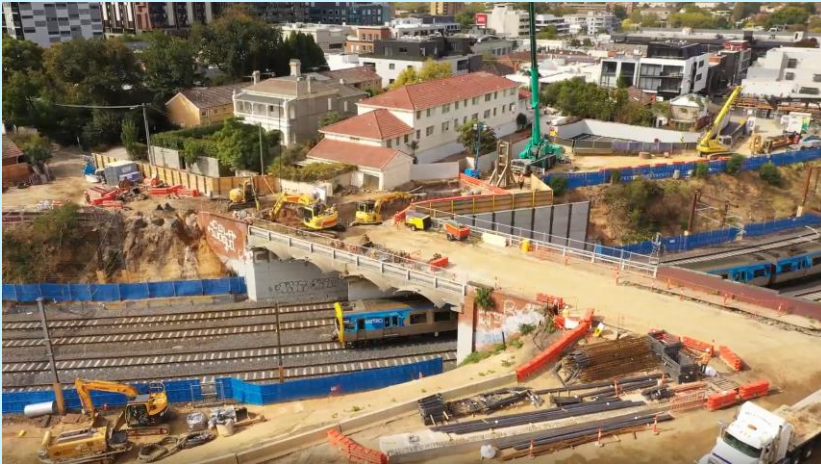
Before – William Street bridge
