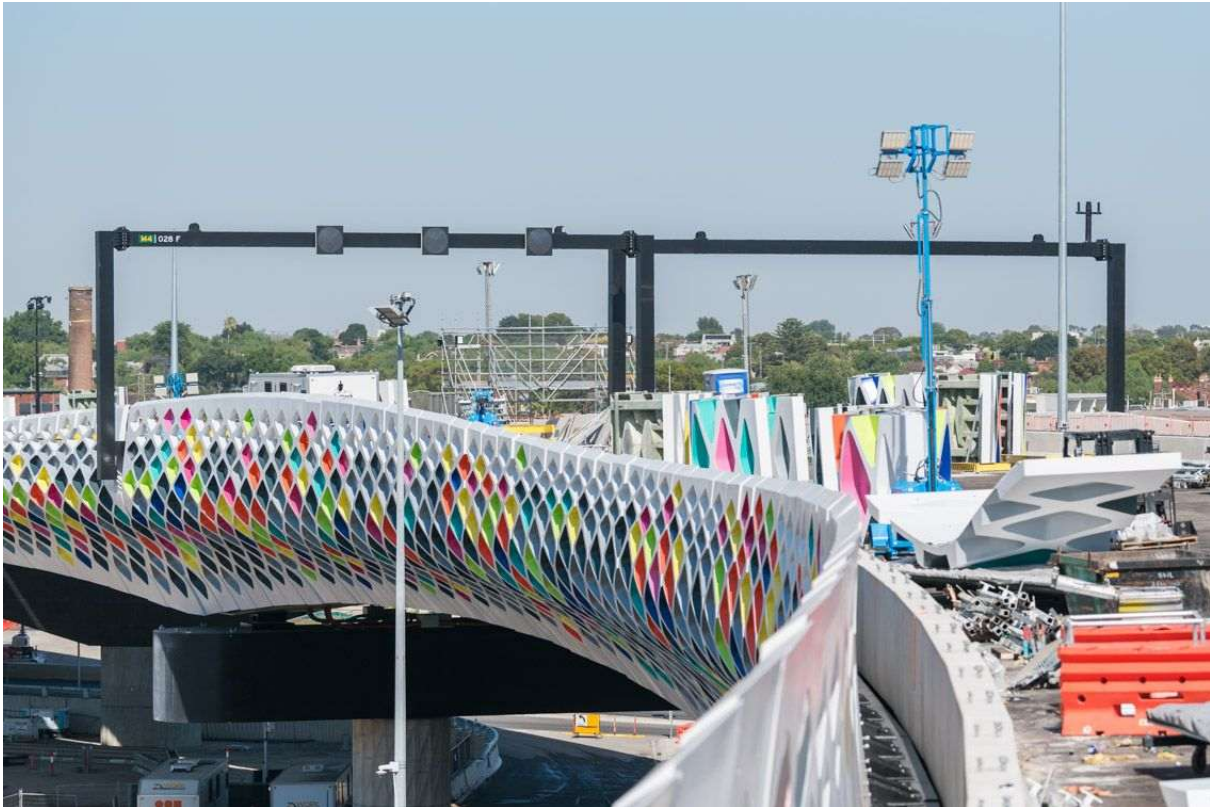
Photo 1 – Eel Skin Cladding, Maribyrnong River Bridge - East Zone (Source: WGTP MRPV, January 2025)
