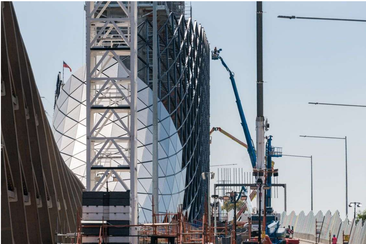
Photo 5 – Southbound Tunnel, Cladding Installation Ventilation Structure (Source: WGTP MRPV, January 2025)
