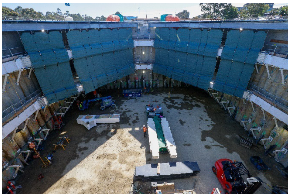
Burwood site progress works, April 2025
