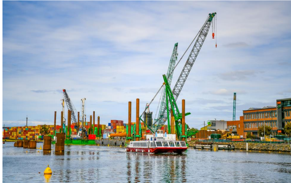
Piling in the Maribyrnong River
