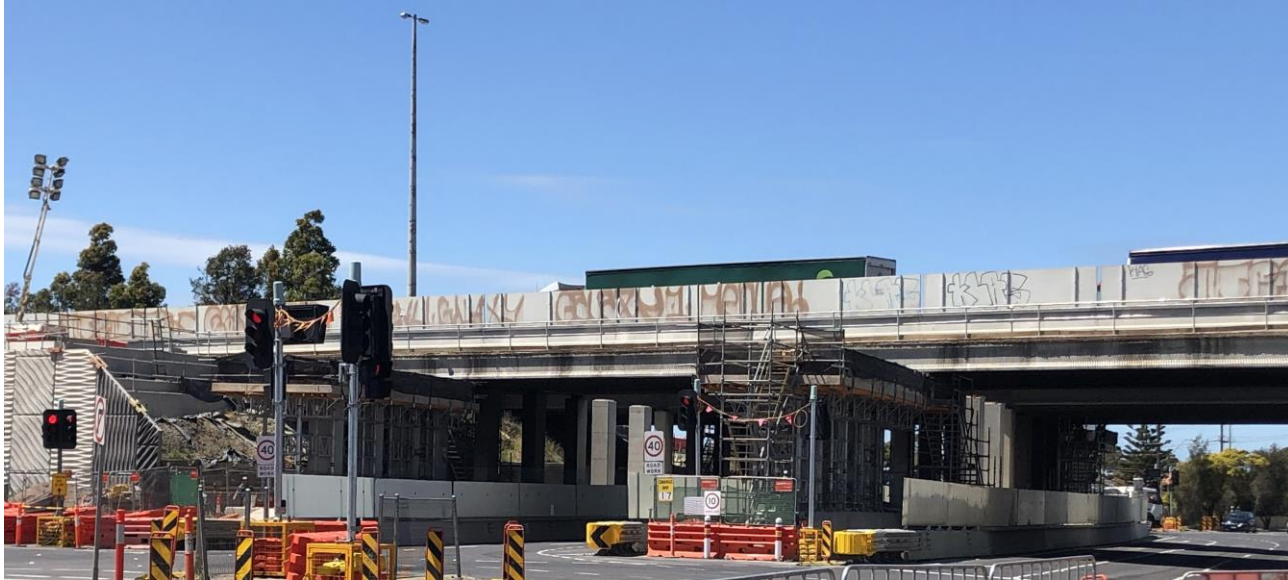
Millers Road interchange
