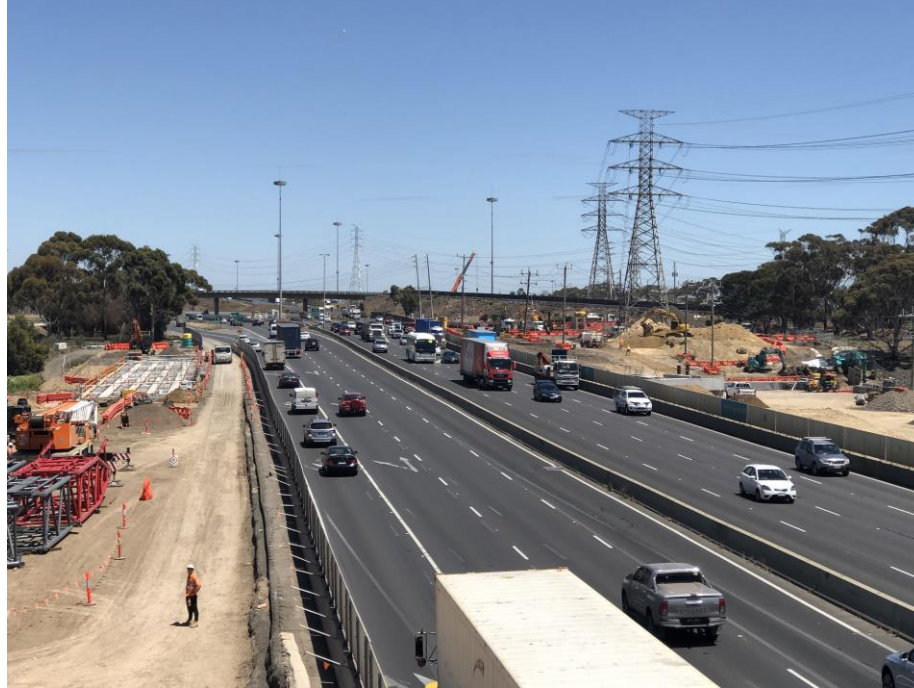
Kororoit Creek Road to M80 interchange - Kororoit Creek Bridge
