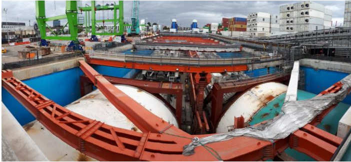
TBM 1 and TBM 2 in launch box
