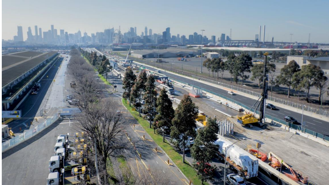
Time lapse of centre median works
