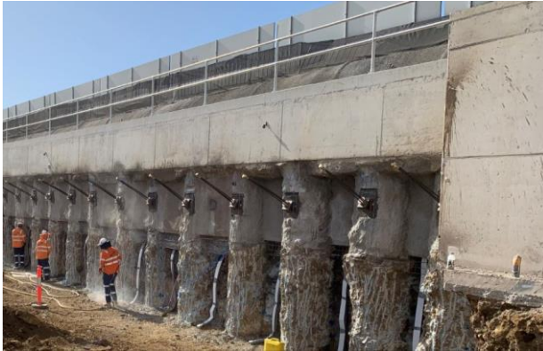
Completed piling works
