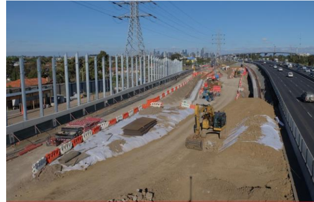
Future tunnel entrance
